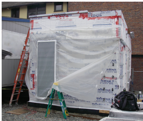
Performance mock-up hut with various representative interfaces and components
