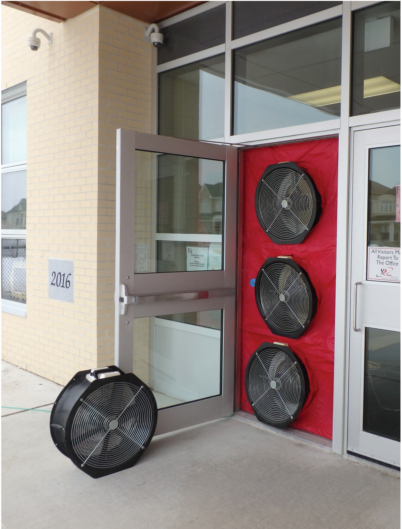
Multiple high-powered blower fans installed in a door opening
