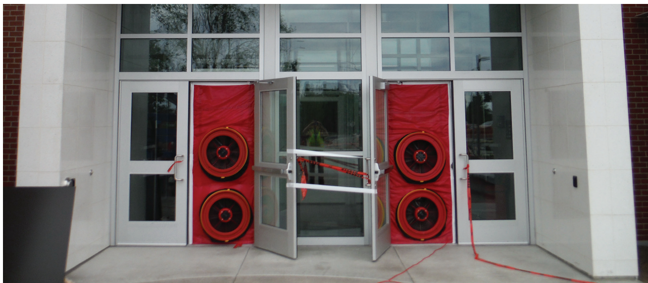
Door fans placed in multiple door openings with frame and fabric enclosures
