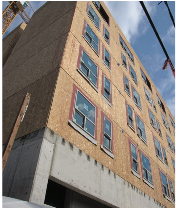
Exterior face of a building with minimal interruptions and interfaces except windows
