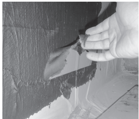
Insufficient adhesion of the membrane likely due to incorrect substrate preparation
