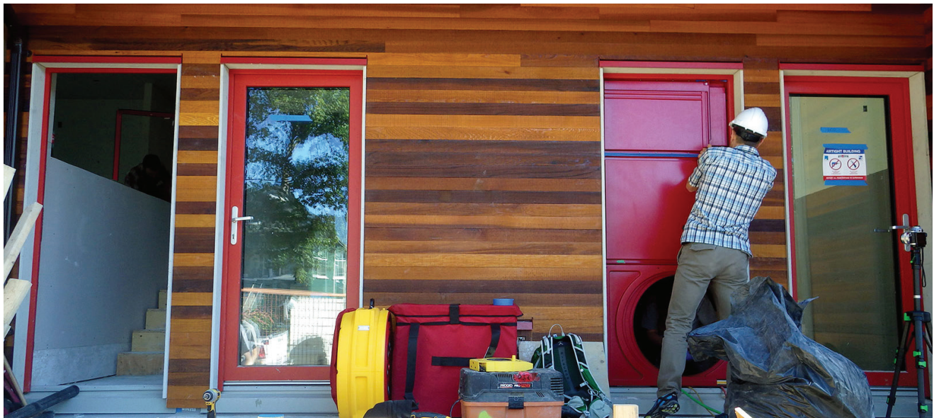
Single door fan to be placed in a door opening using a solid enclosure
