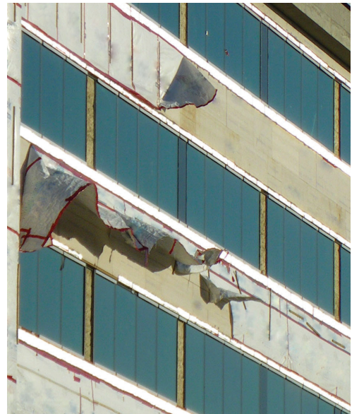
Damaged air barrier during construction
