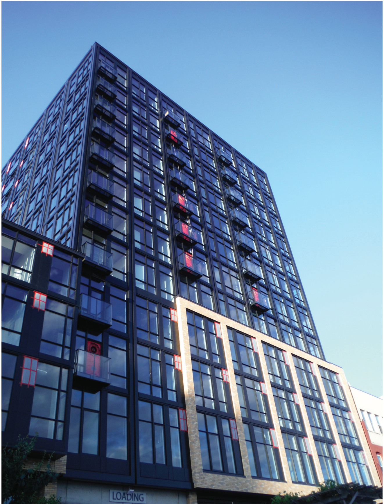
Quantitative airtightness testing with multiple fans on a large building occurring near the end of construction
