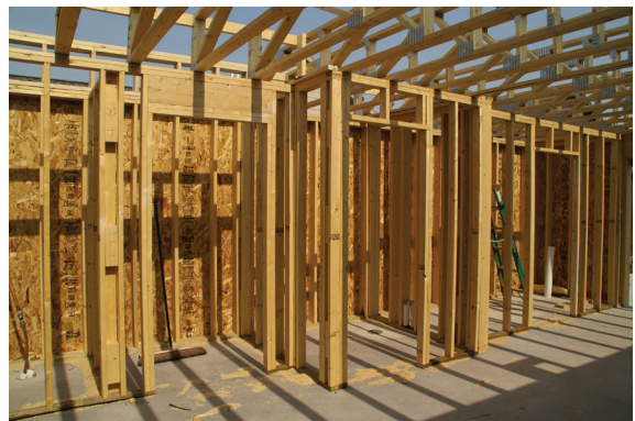
Wall framing and floor assembly interfacing with the exterior wall assembly at the interior side
