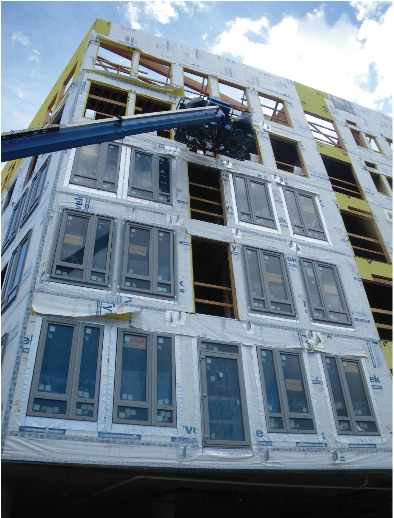
Wood-frame building over concrete podium, designed to allow completion of the air barrier before balconies are installed on clips
