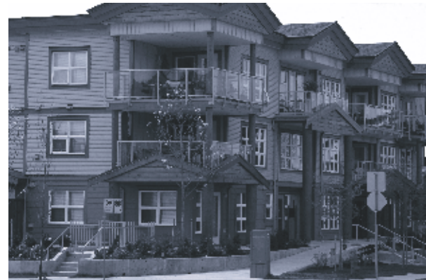
Lu'ma Native Housing development, located in Vancouver, provides 22 units of mixed income housing for Aboriginal families and singles.
