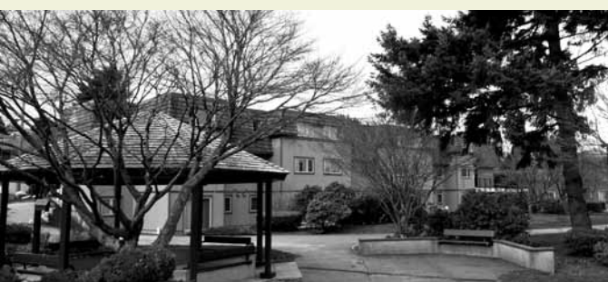
Extensive renovations and energy retrofits have extended the life of Stratford Gardens by at least 30 years.
