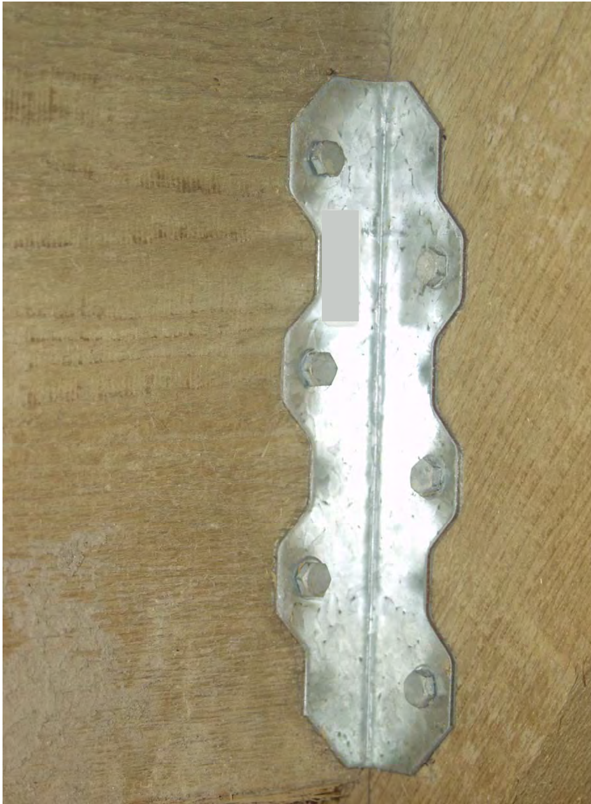
Figure 43. Galvanized connectors showing red rust on the edge. Note lack of watermarking of timber
