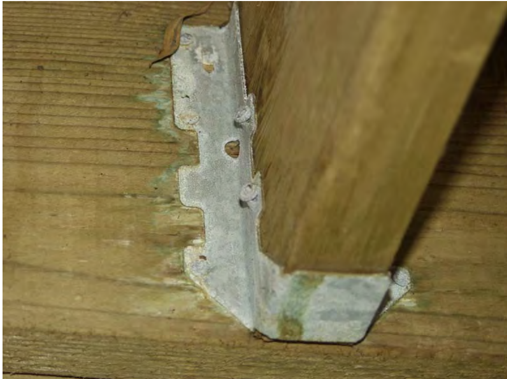
Figure 10 Copper deposits and red rust on lower edge of hanger
