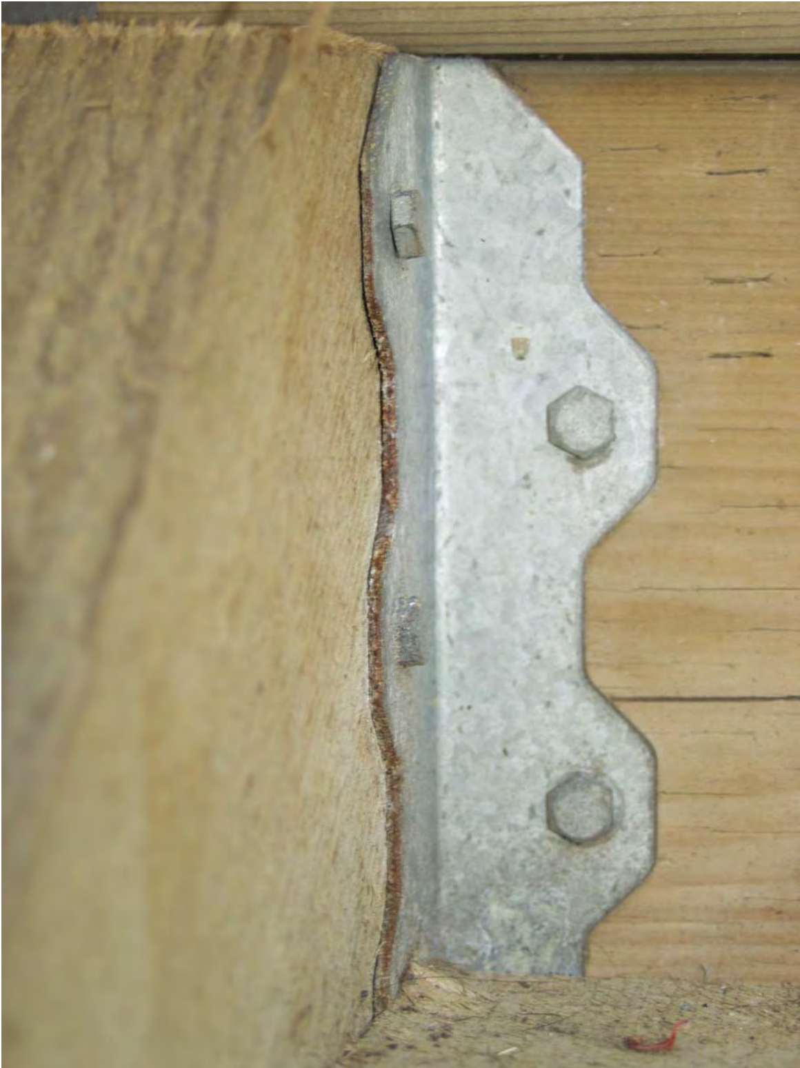
Figure 45 Galvanized connectors showing red rust on the edge. Note lack of watermarking of timber
