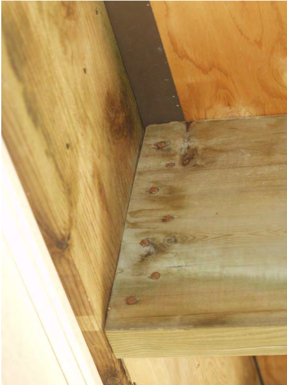
Figure 20. Red rust on nails fastening deck joist to rim joist. Blocking is used in this design so no hangers are required
