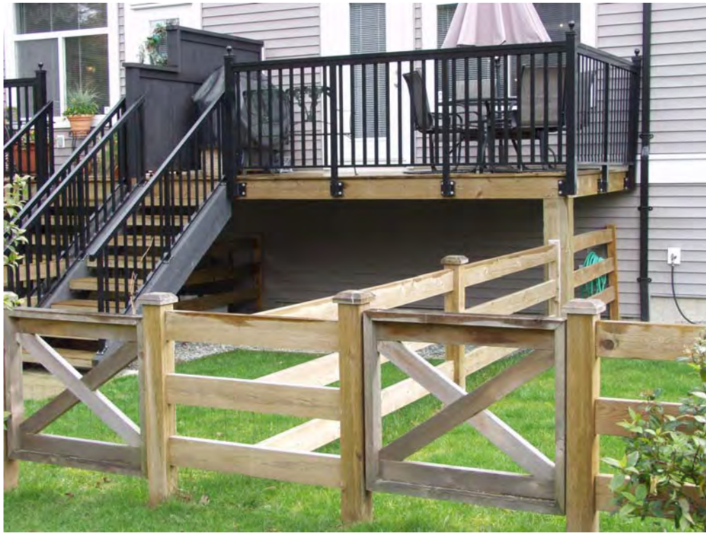
Figure 1 General view showing treated wood fence and decks
