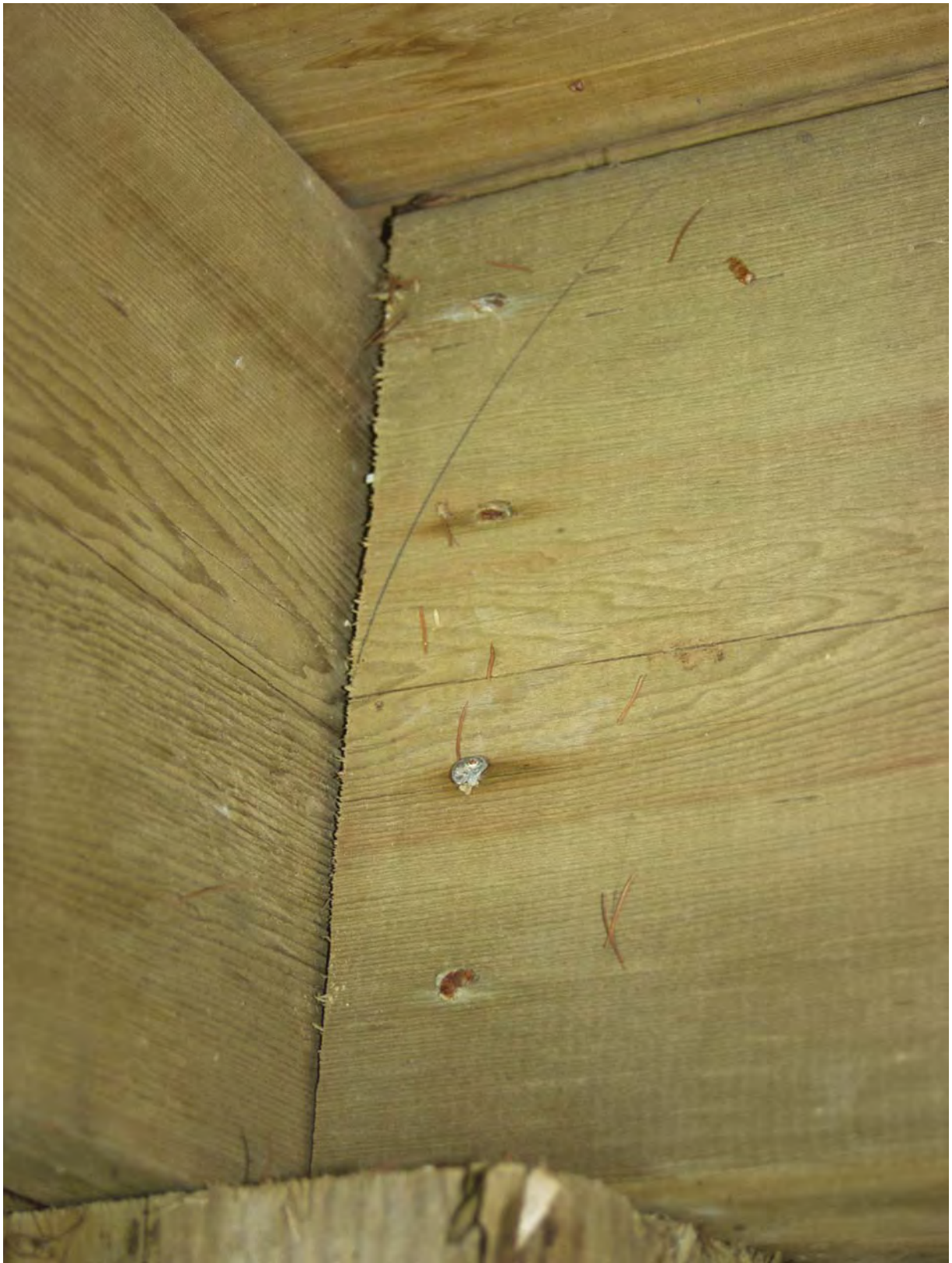
Figure 39. Galvanized fasteners showing red rust on their heads due to loss of zinc during nailing
