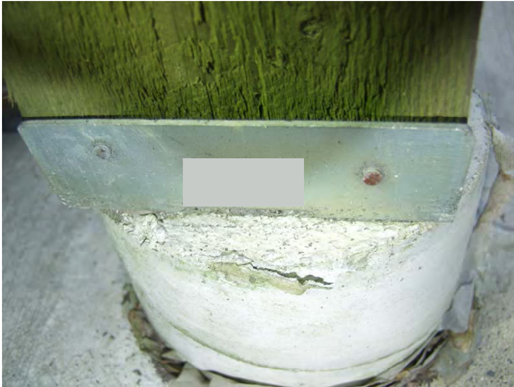
Figure 53. Galvanized post base connector showing no corrosion. Galvanized fastener heads show red rust due to loss of zing during nailing
