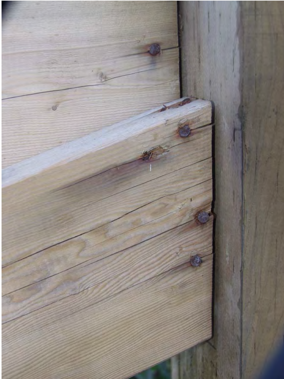
Figure 25. Red rust on un-galvanized nails.
