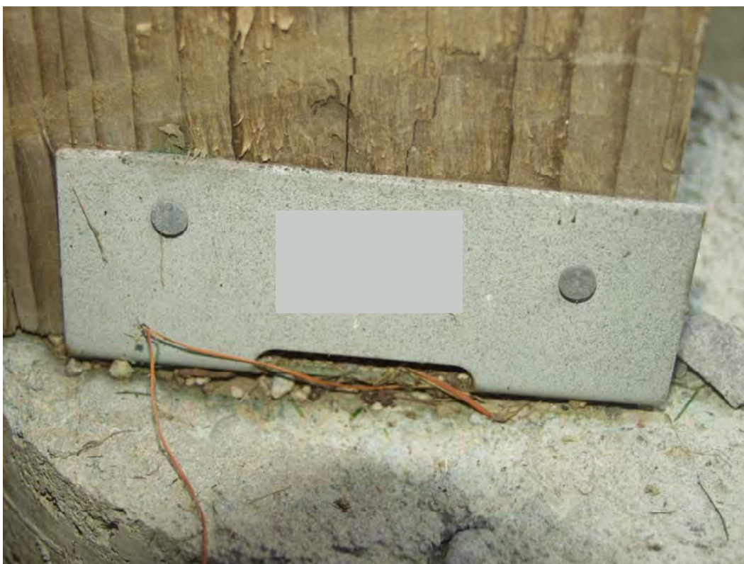
Figure 32. Galvanized connector and nails for post base showing no corrosion
