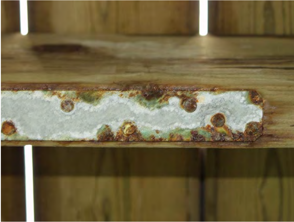
Figure 5 Electroplated strapping showing red rust
