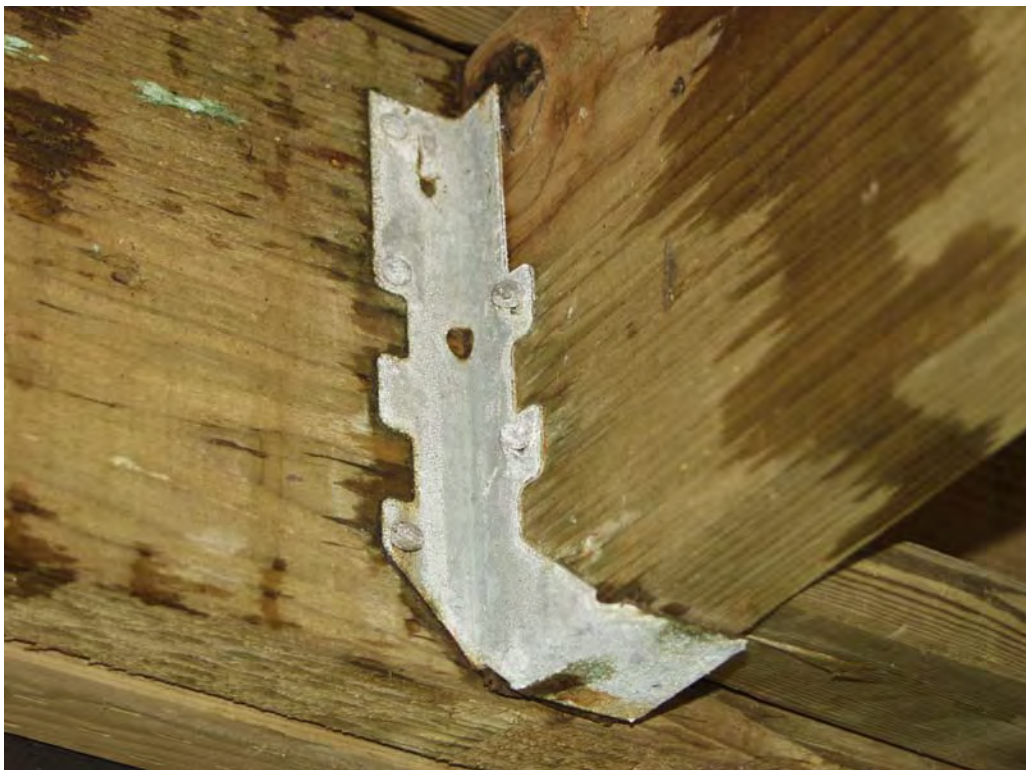
Figure 11 Copper deposits and red rust on edges of hanger and nails
