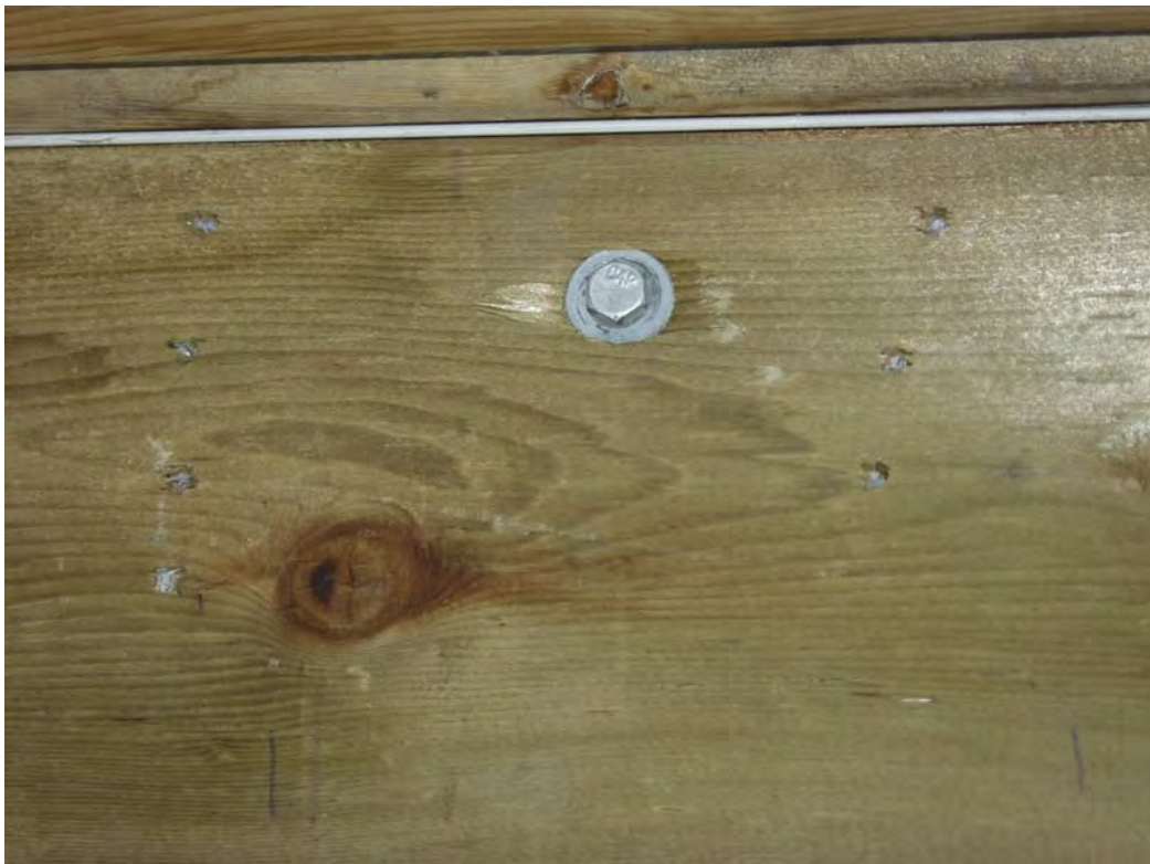
Figure 37. Galvanized bolt, washer and nails in unincised ACQ deck joist show no corrosion
