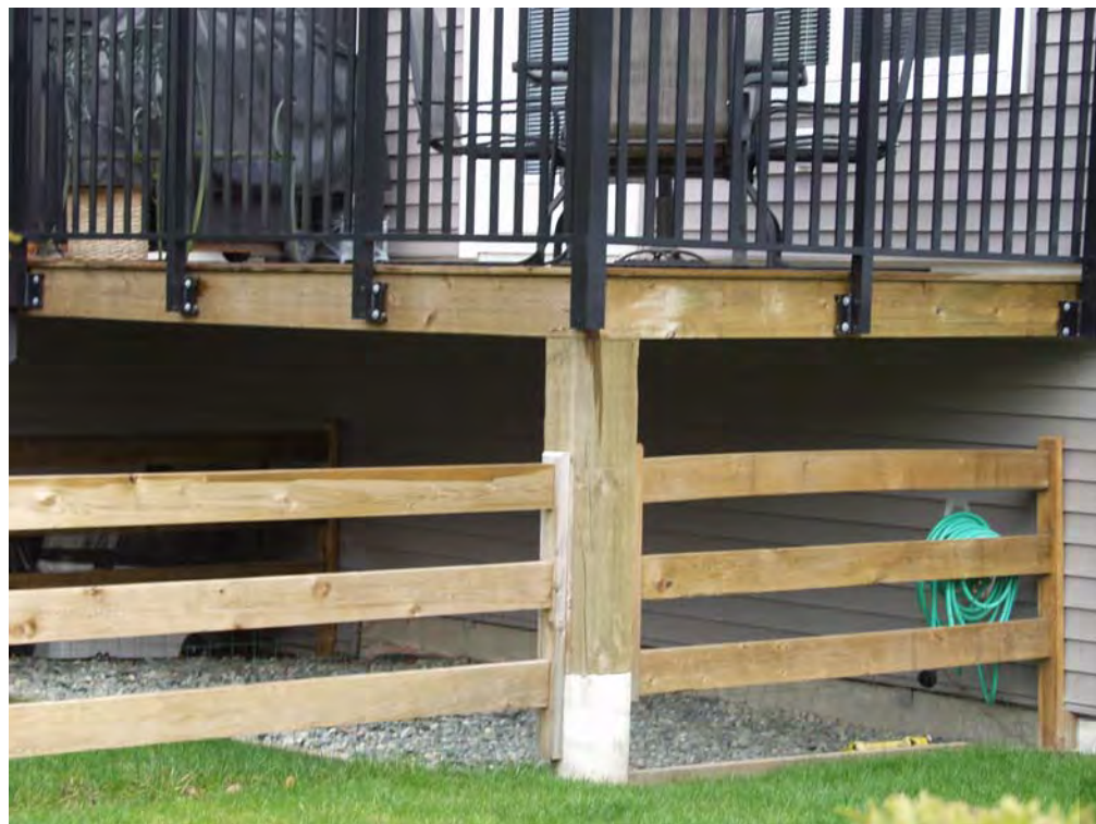
Figure 2 General view showing treated decks
