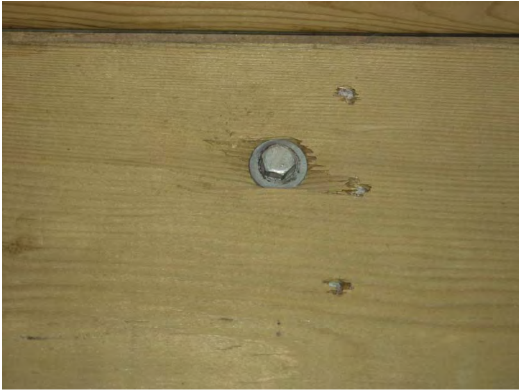
Figure 36. Galvanized bolt, washer and nails in unincised ACQ deck joist show no corrosion
