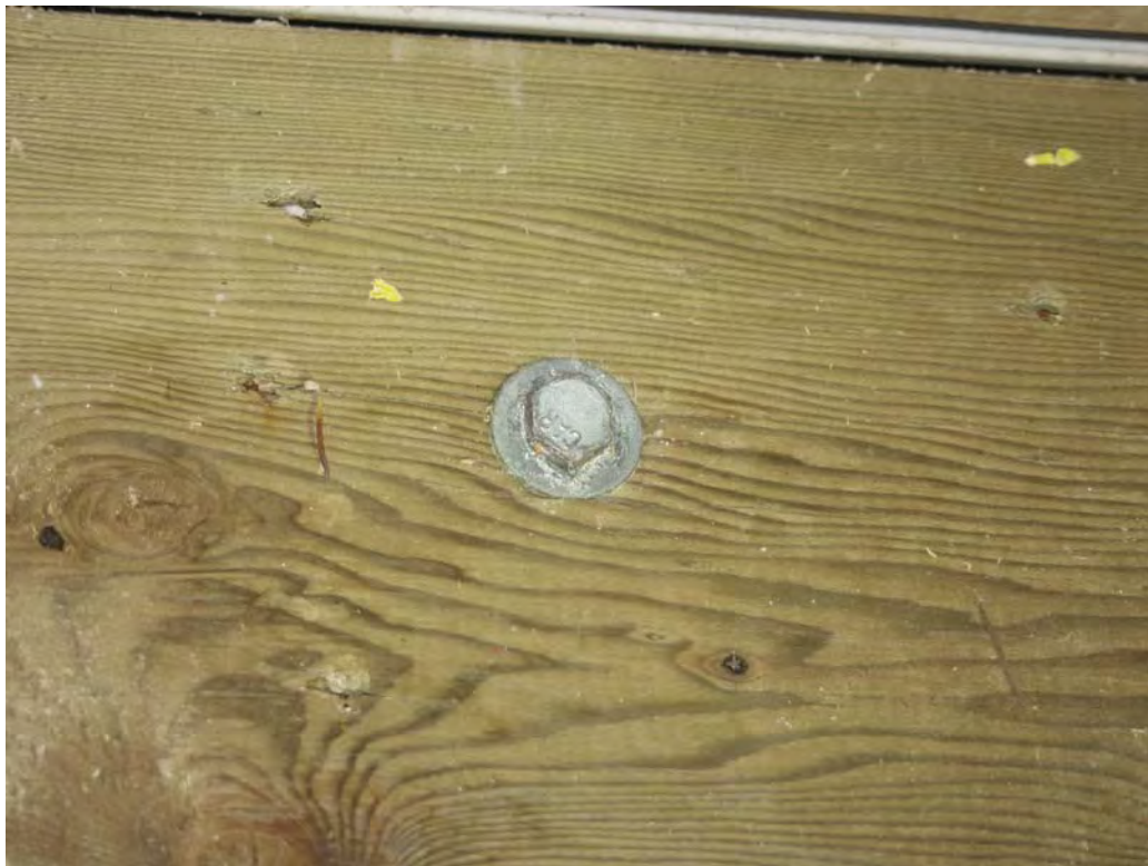
Figure 30. Bolt, washer and nails all free from corrosion
