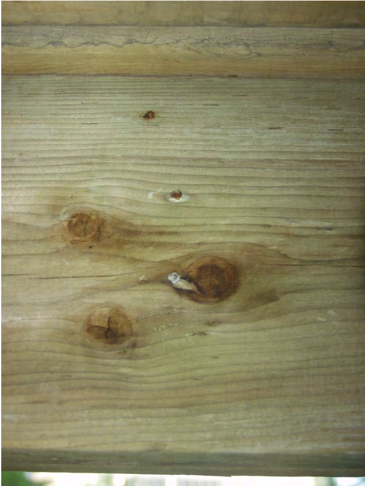
Figure 40. Galvanized fasteners showing red rust on their heads due to loss of zinc during nailing in incised ACQ lumber
