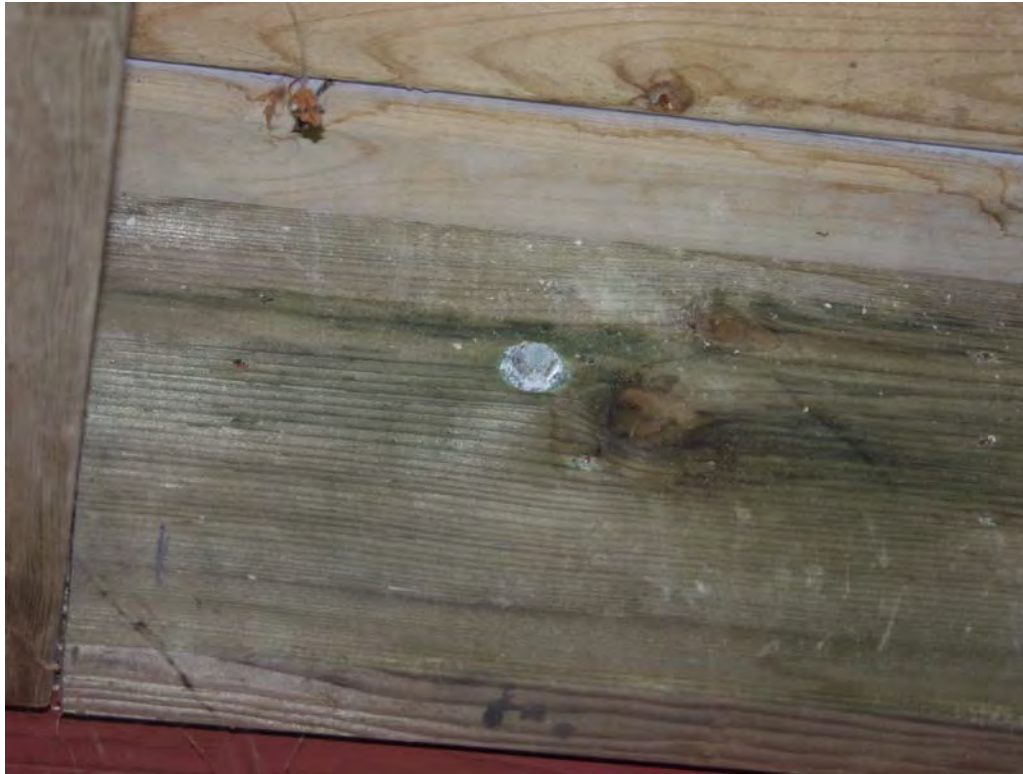
Figure 29. White rust on galvanized bolt
