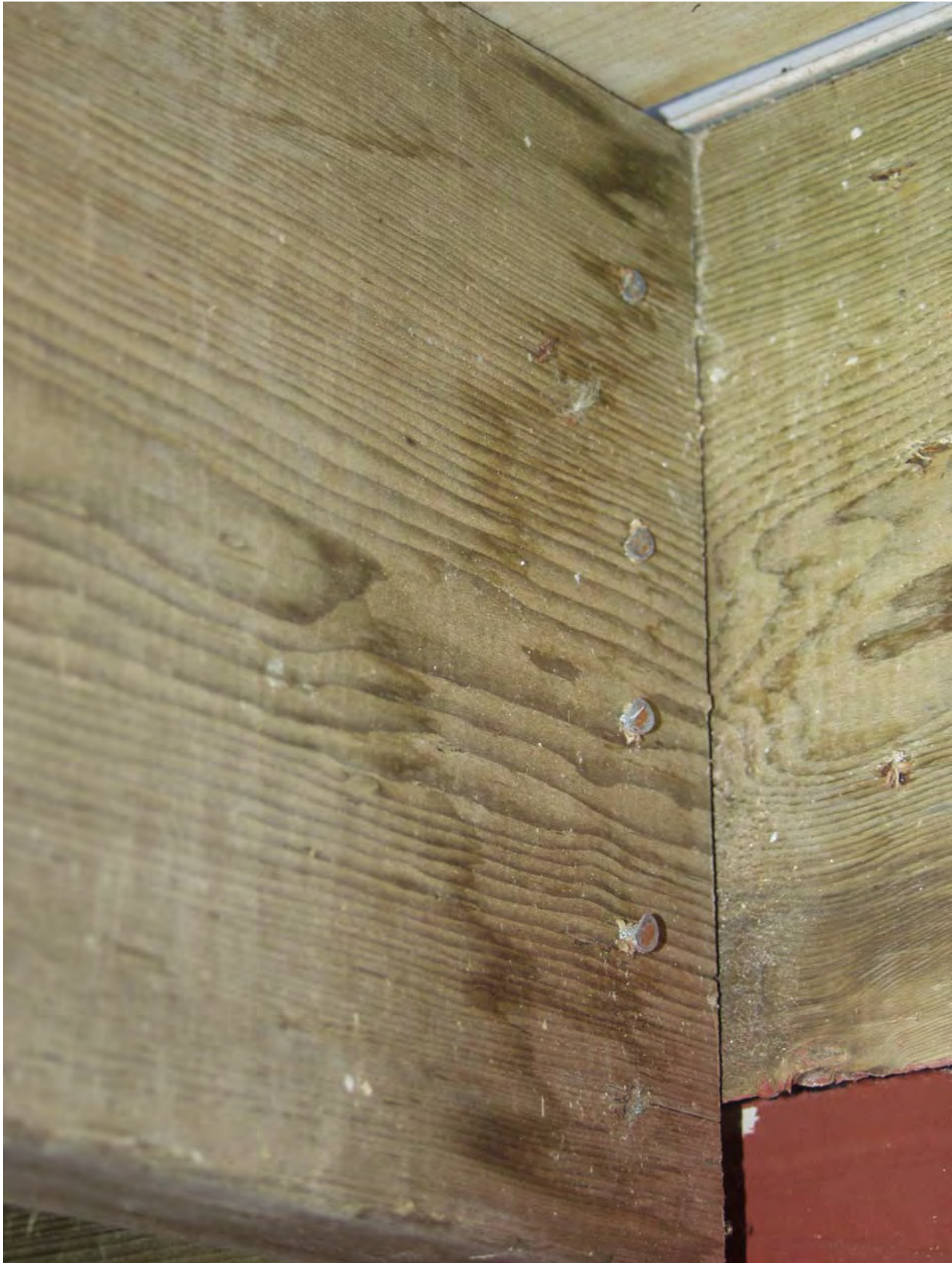
Figure 34. Galvanized nails in unincised ACQ deck joist show corrosion (red rust) on the heads most probably due to loss of zinc coating during nailing.
