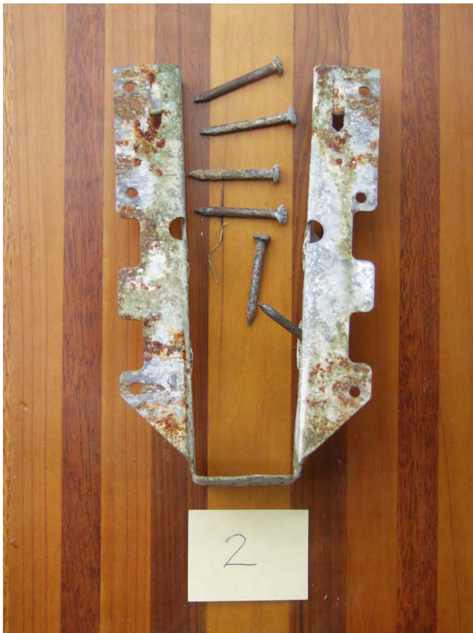
Figure 60. Corrosion of hot dipped galvanized hanger proprietary hanger, (the specifications of which meets the G185 requirement) and fasteners after 11 months exposure.
