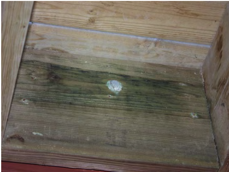
Figure 27. White rust on galvanized bolt
