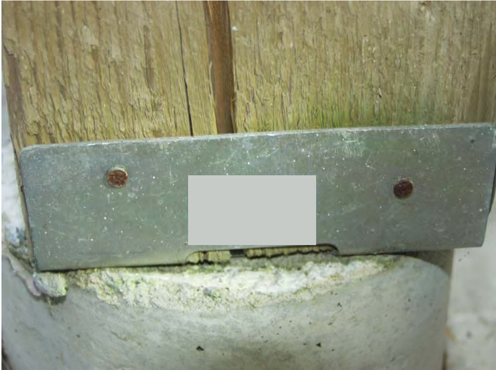
Figure 55. Galvanized post base connector showing no corrosion. Galvanized fastener heads show red rust due to loss of zing during nailing
