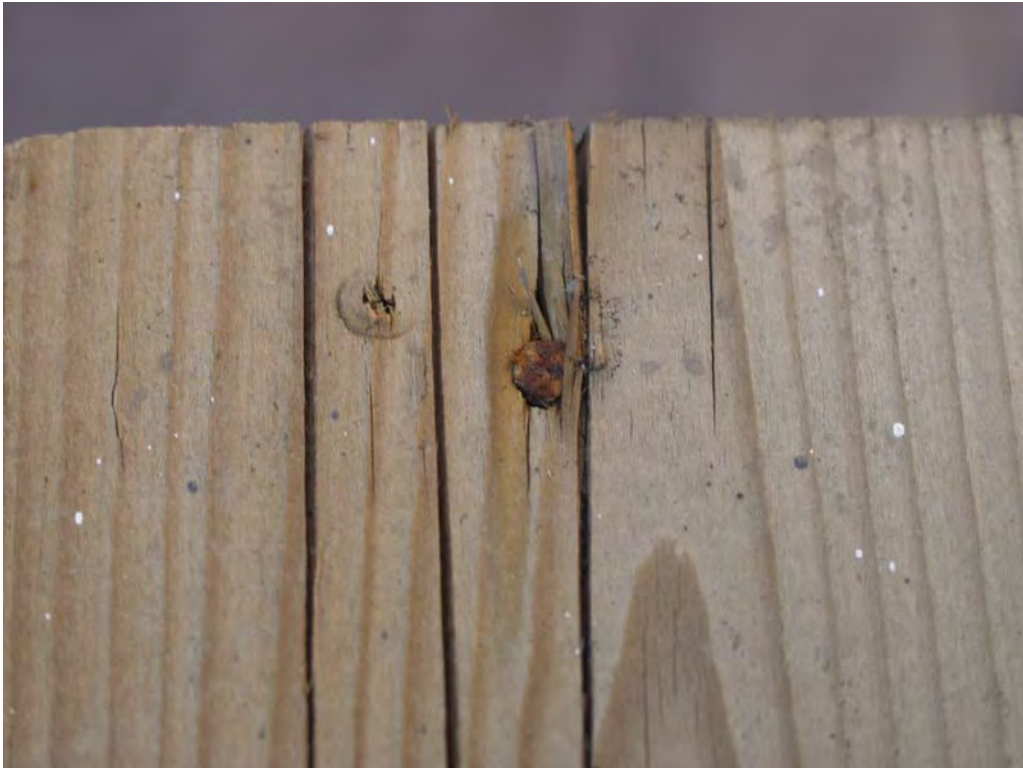
Figure 22. Red rust on common mild steel nails fastening stairs.
