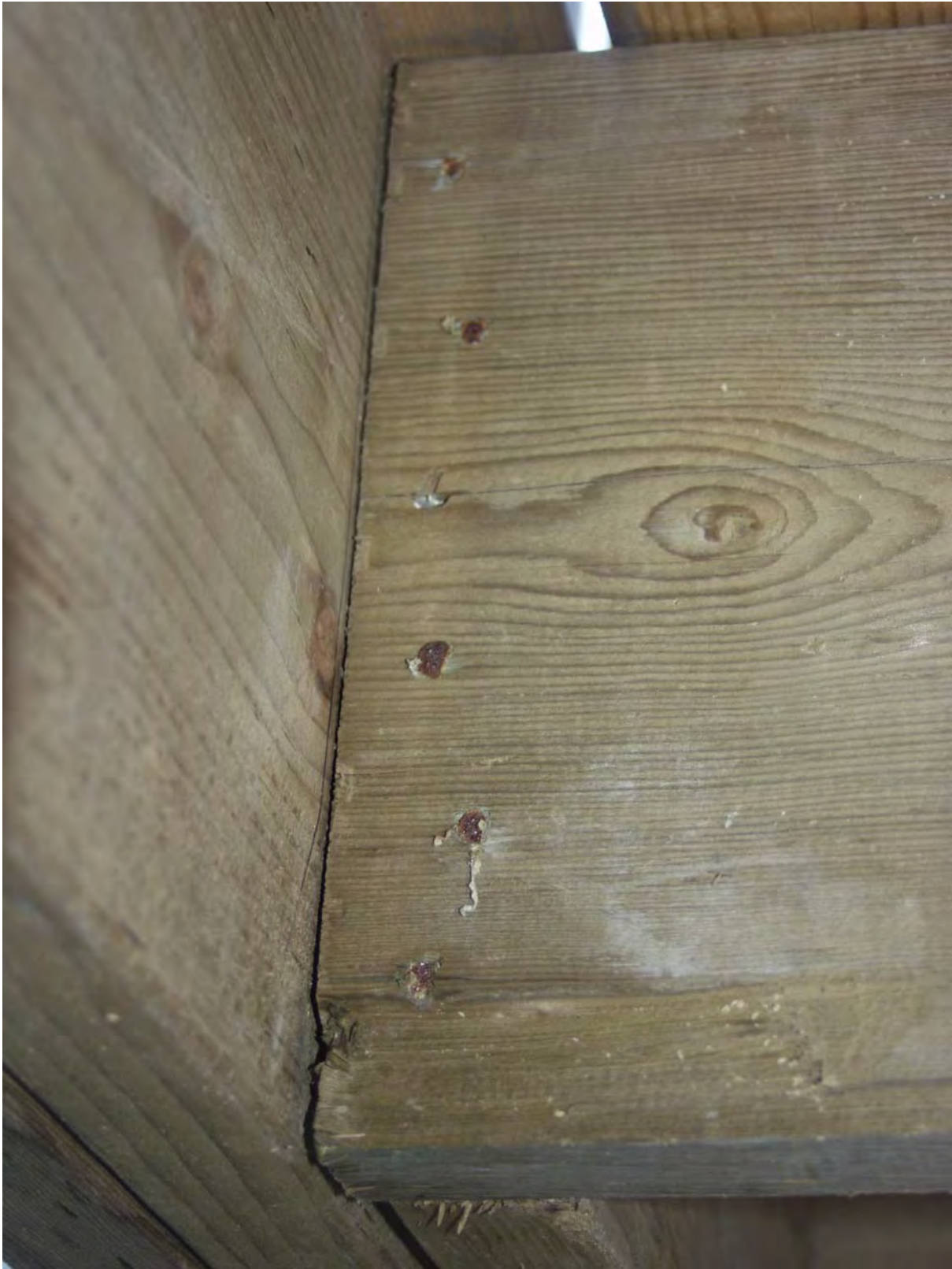
Figure 35. Galvanized and possible common nails in unincised ACQ deck joist show corrosion (red rust) on the heads. Note lack of water marking on lumber.
