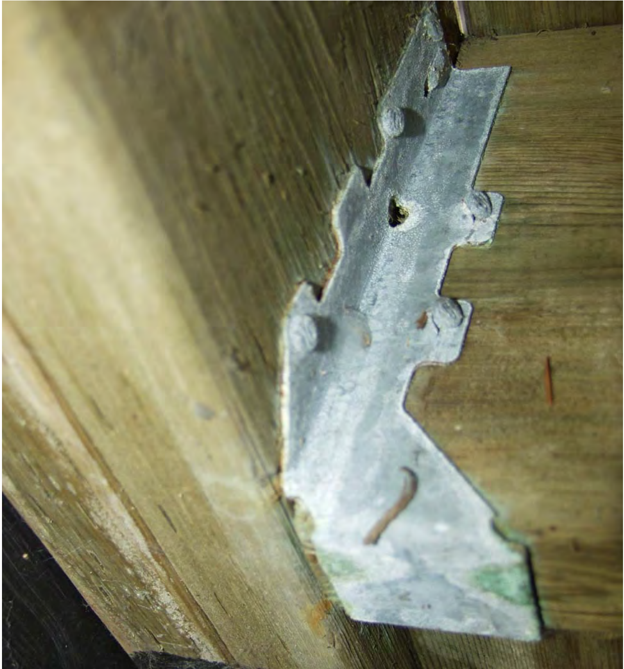
Figure 16 White rust on proprietary hanger, (the specifications of which meets the G185 requirement) and nails. Green copper deposit visible on lower hanger surface.
