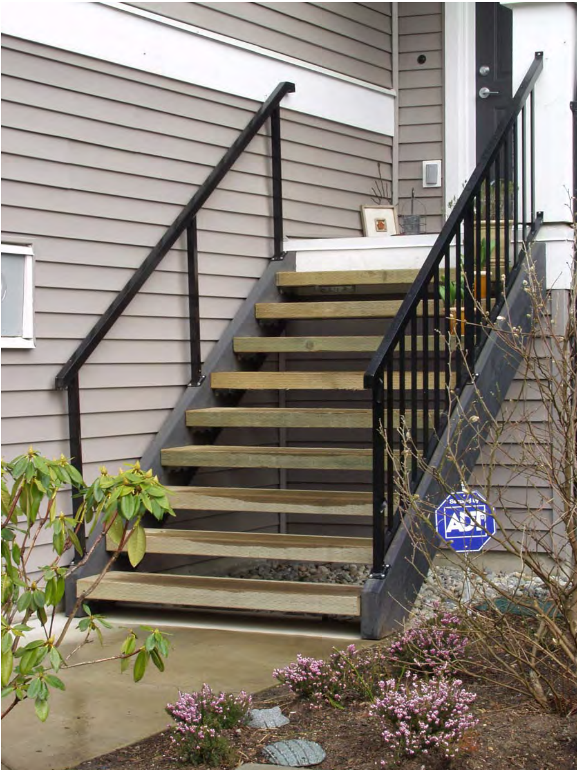
Figure 9 Stairs showing construction design
