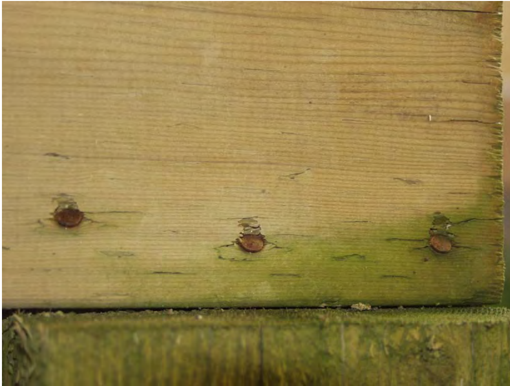
Figure 48. Corrosion (red rust) on mild steel fasteners in contact with incised ACQ treated wood.
