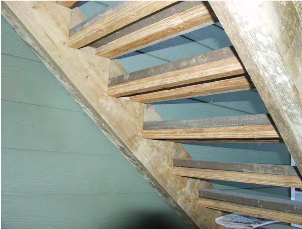
Figure 41. Design of stairs showing untreated oriented strand lumber separating plastic tread from ACQ lumber
