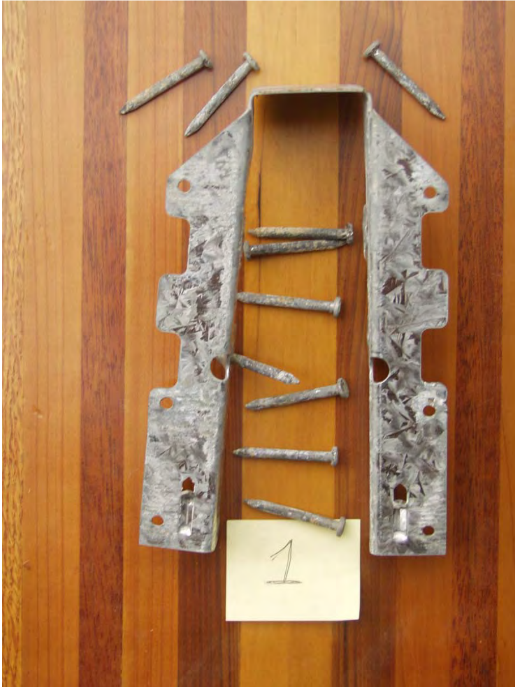
Figure 58. Galvanized hanger the specifications of which meet the G 185 requirement removed from deck protected from weather.
