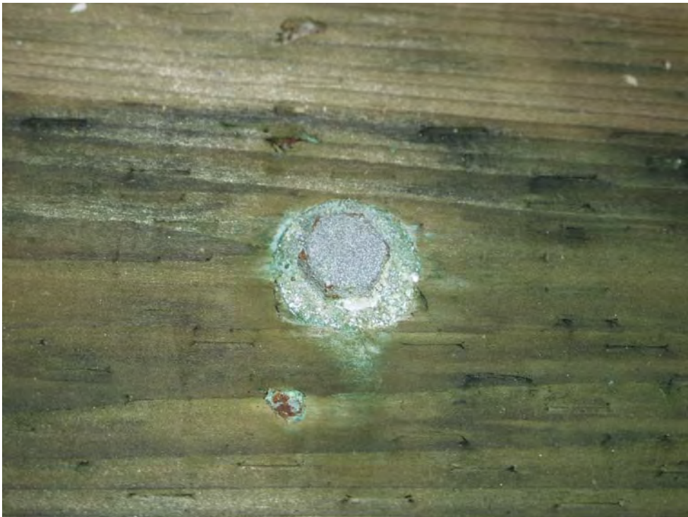
Figure 28. White rust on galvanized bolt and washer contacting incised ACQ treated wood
