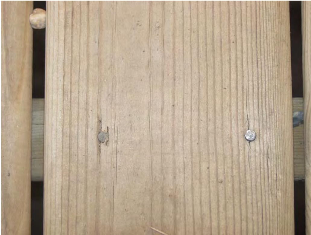
Figure 47. Galvanized fasteners on decking – no corrosion visible
