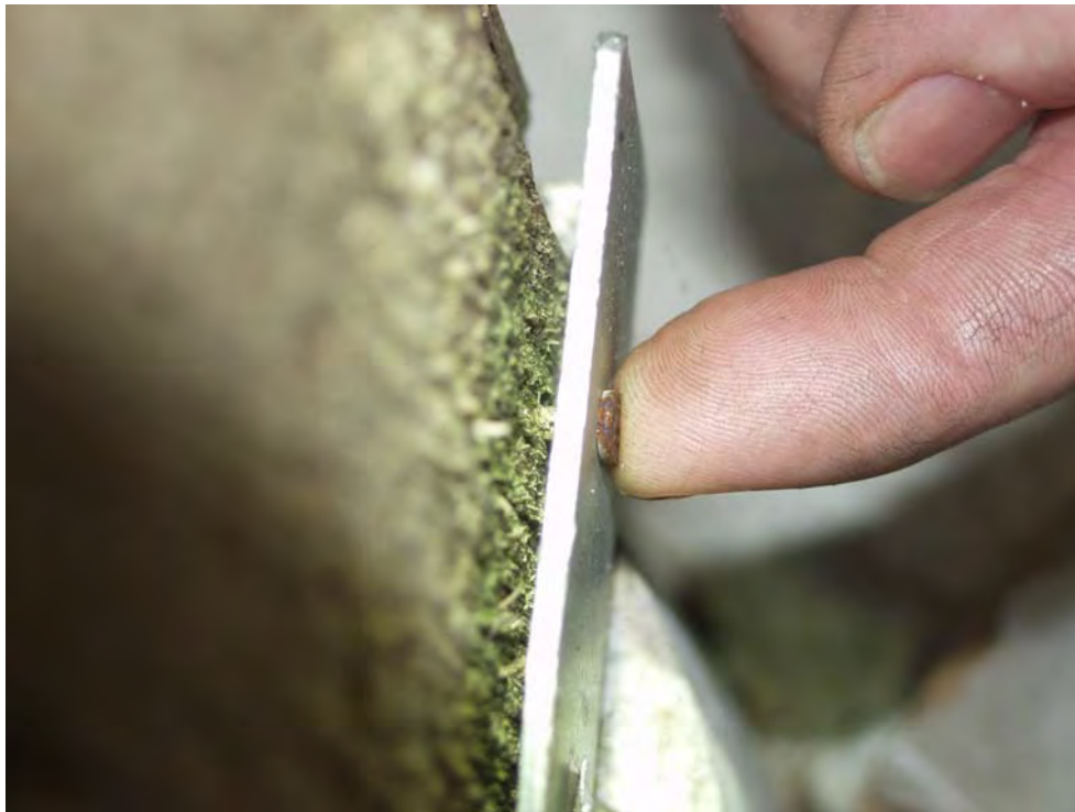
Figure 52. Galvanized fastener show white and red rust due to loss of zing during nailing
