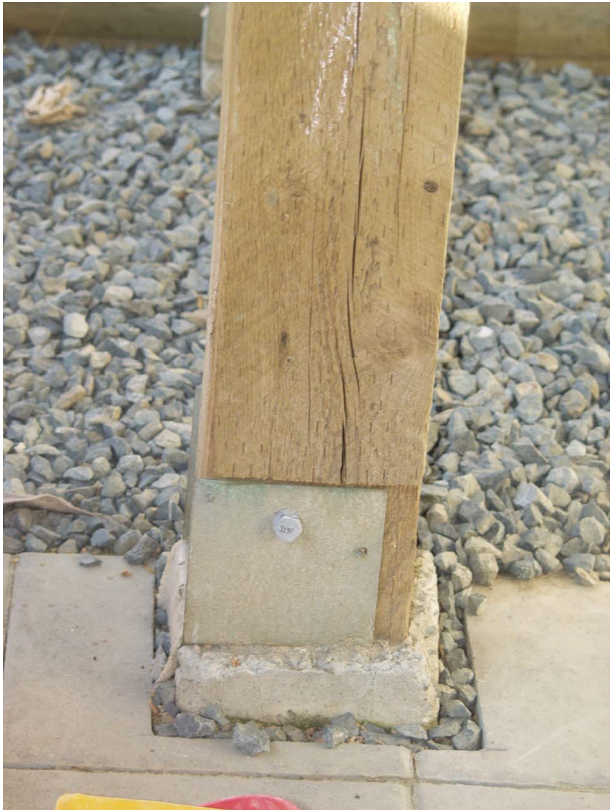
Figure 19 Post support showing absence of corrosion
