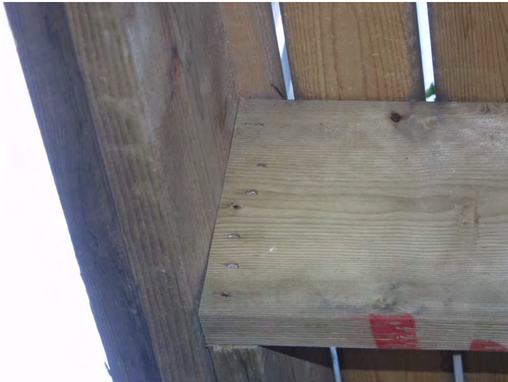
Figure 31. Red rust on common mild steel nails
