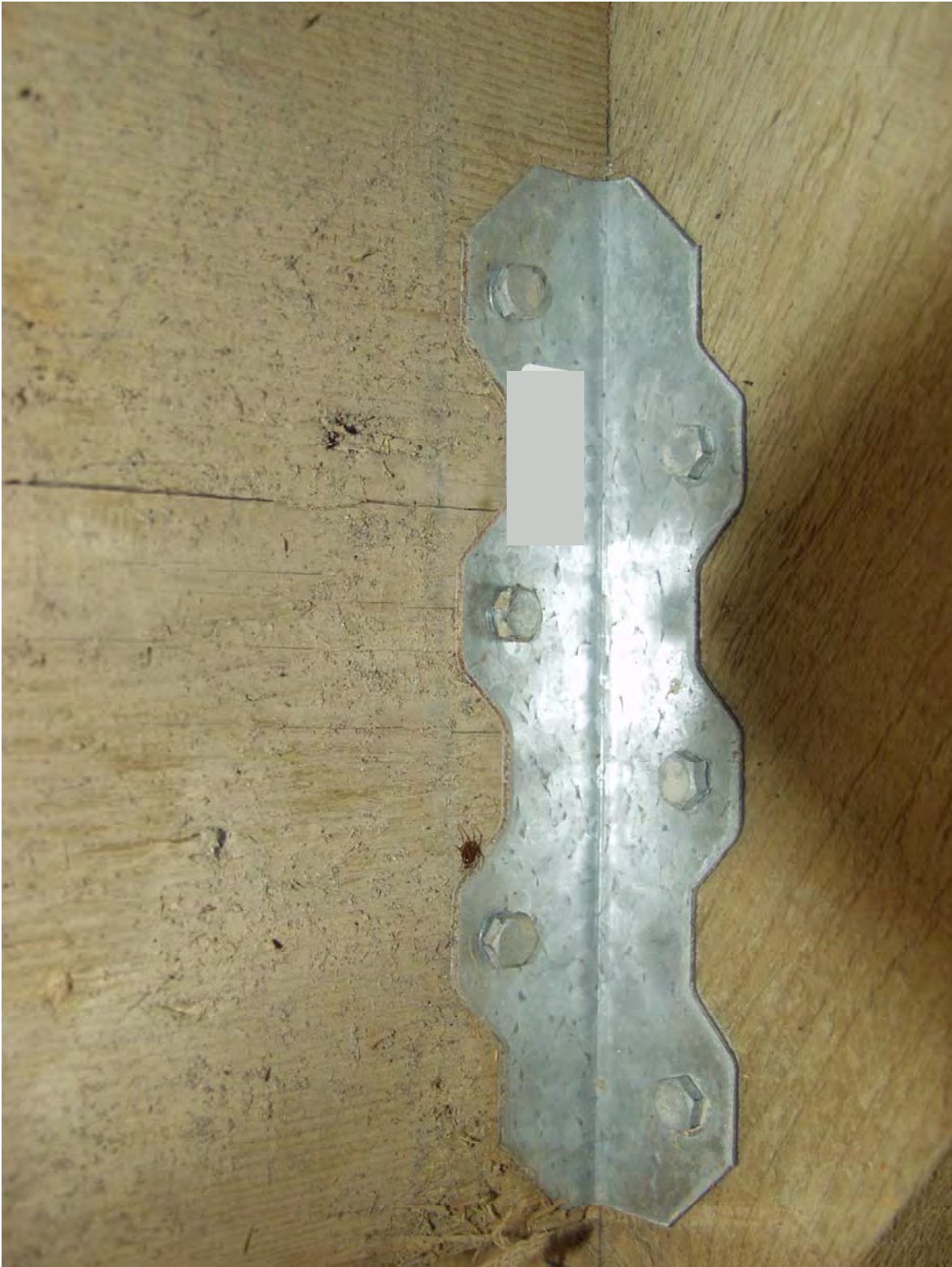
Figure 44. Galvanized connectors showing red rust on the edge. Note lack of watermarking of timber
