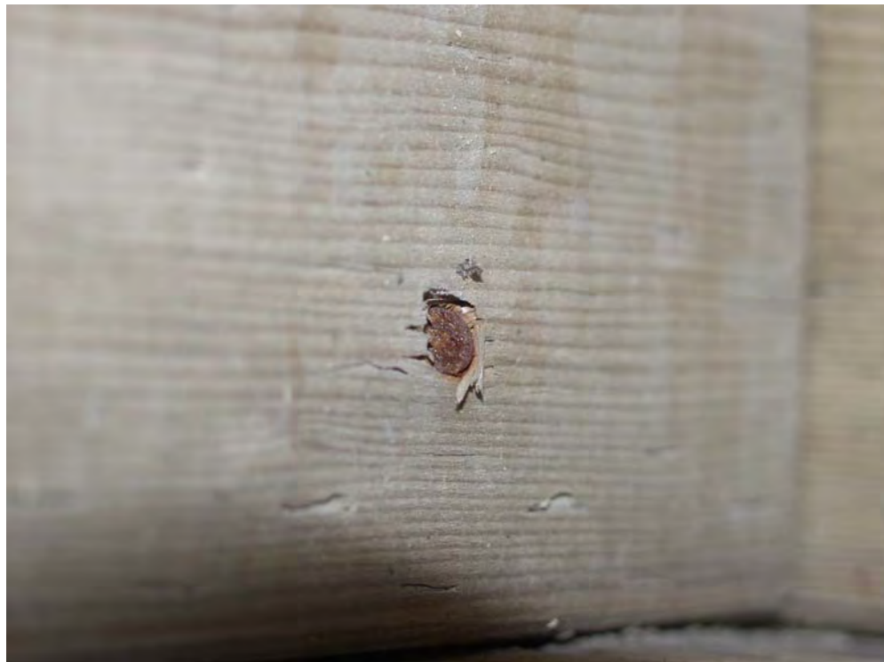
Figure 50. Corrosion (red rust) on the head of common (mild steel) fasteners in contact with unincised ACQ treated lumber
