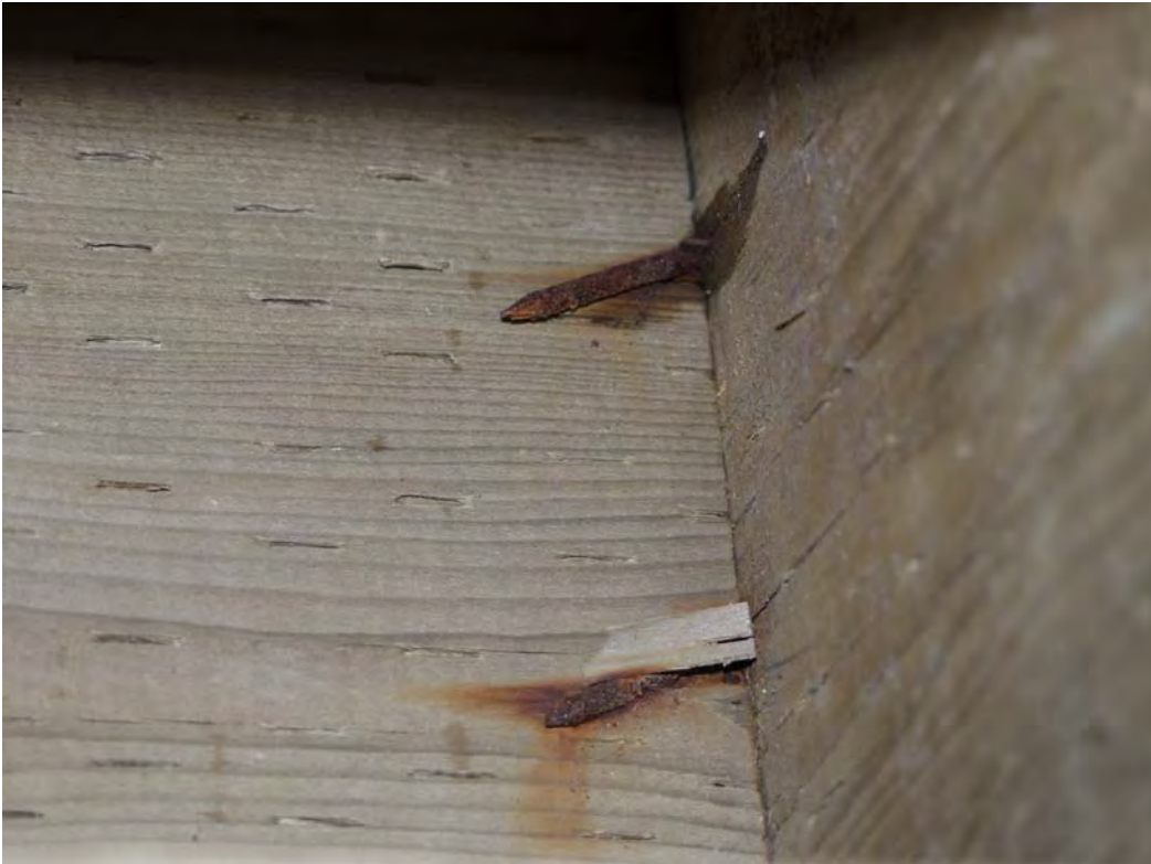
Figure 7 Corrosion of mild steel un-galvanized nails
