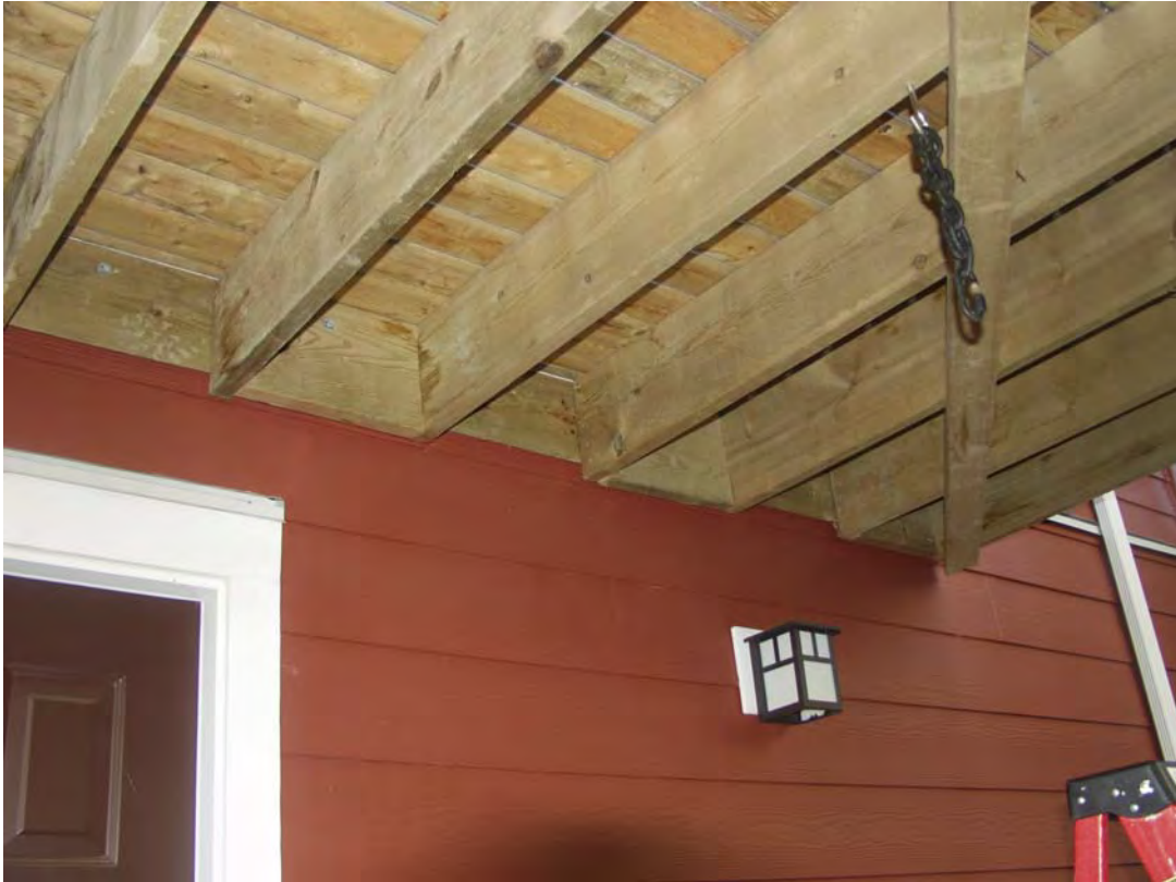
Figure 38. Design of decking showing blocking. No hangers were used in this design.
