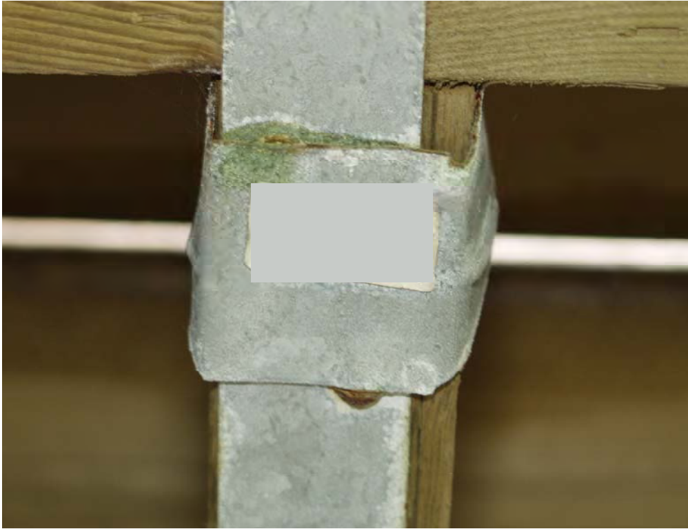
Figure 3 Hanger with red rust and copper deposits
