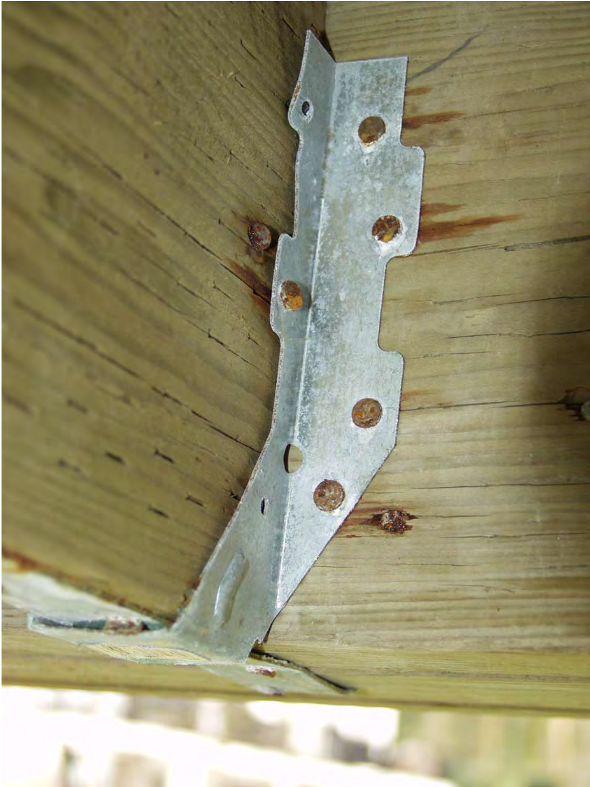
Figure 6 Red rust on common fasteners
