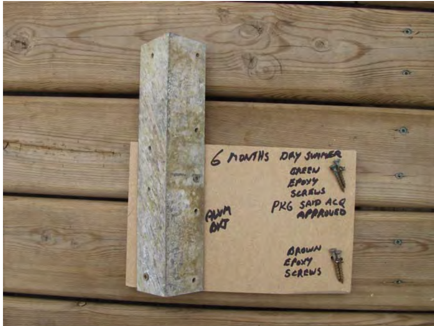
Figure 56. Corrosion of aluminum bracket and decking screws after 6 months service in ACQ decking
