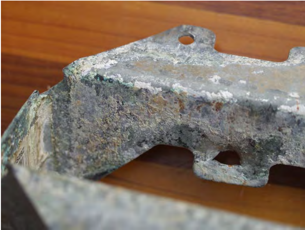
Figure 61. Corrosion of proprietary hot dipped galvanized hanger, (the specifications of which meets the G185 requirement) after 11 months exposure in contact with ACQ treated wood.
