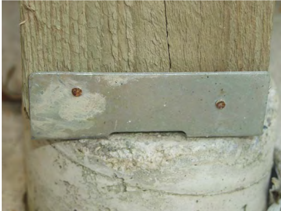
Figure 51. Galvanized post base connector showing no corrosion. Galvanized fastener heads show red rust due to loss of zing during nailing
