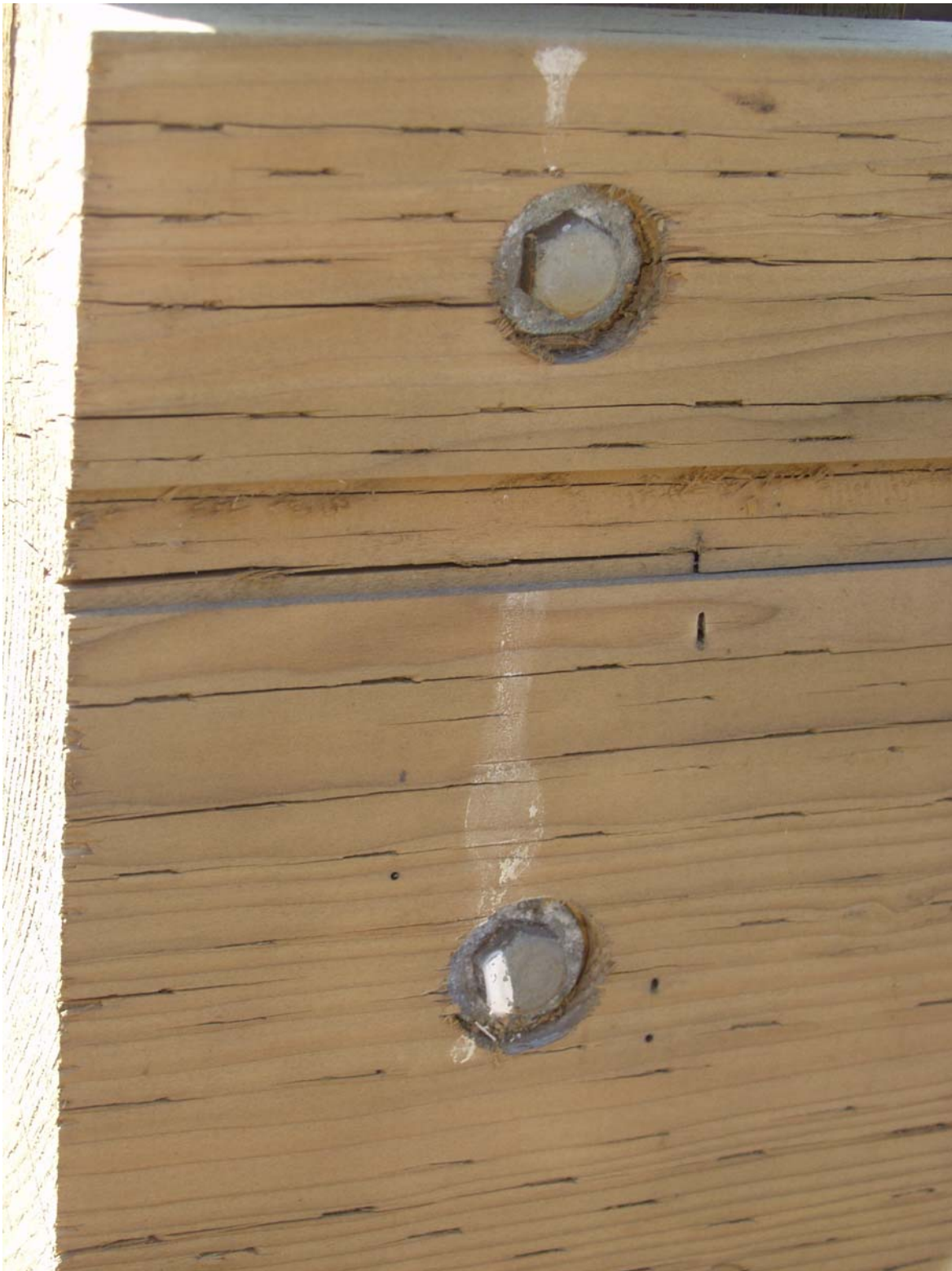
Figure 26. Corrosion on bolts on barrier fencing made from ACQ treated wood
