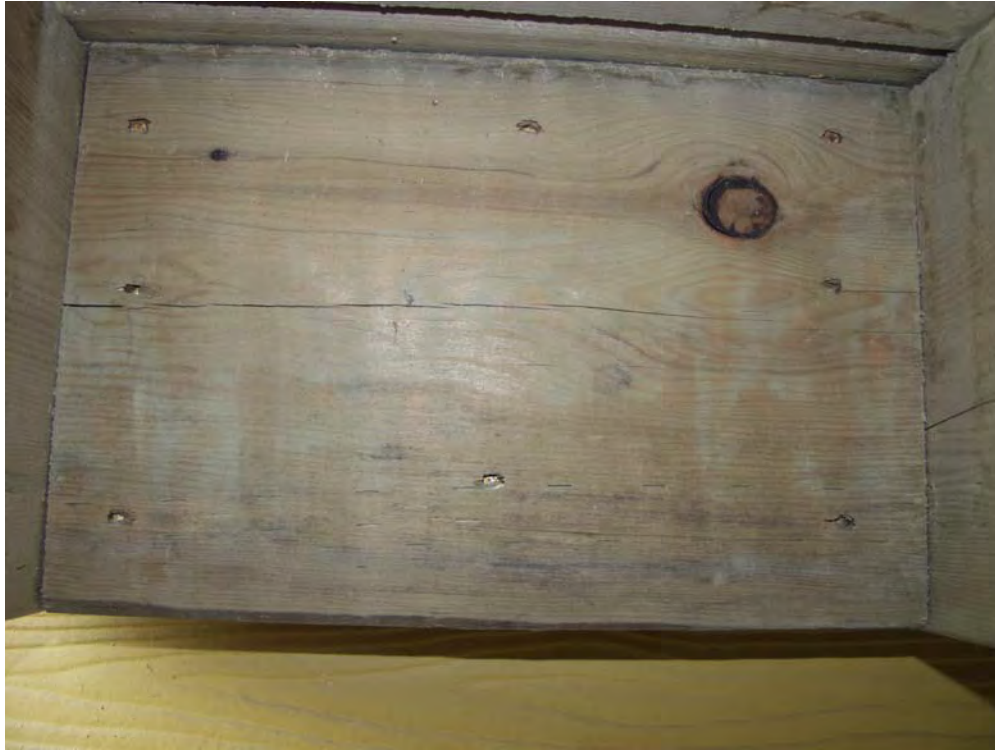
Figure 49. Galvanized fasteners showing no corrosion
