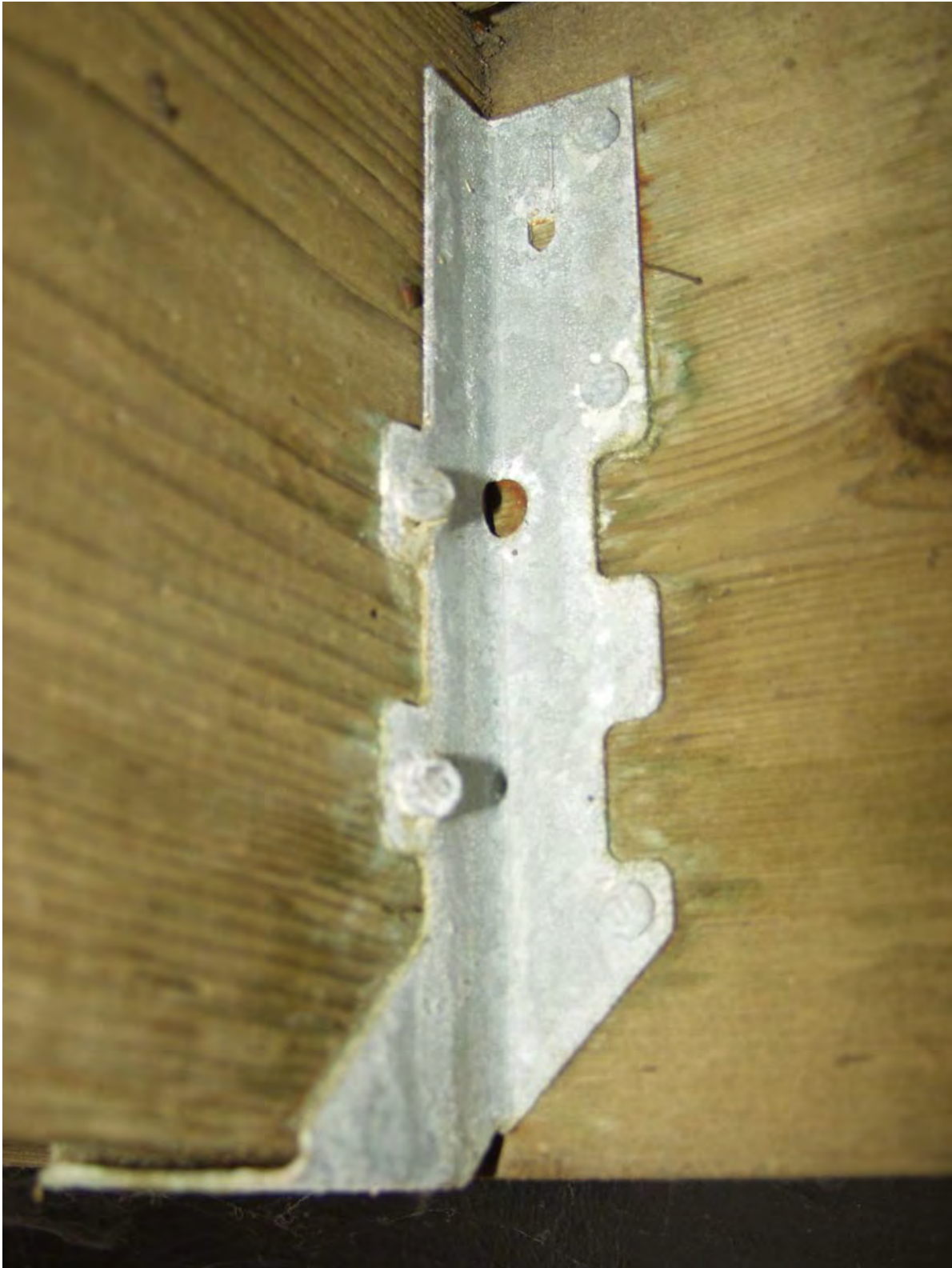
Figure 15 White rust on proprietary hanger, (the specifications of which meets the G185 requirement) and nails
