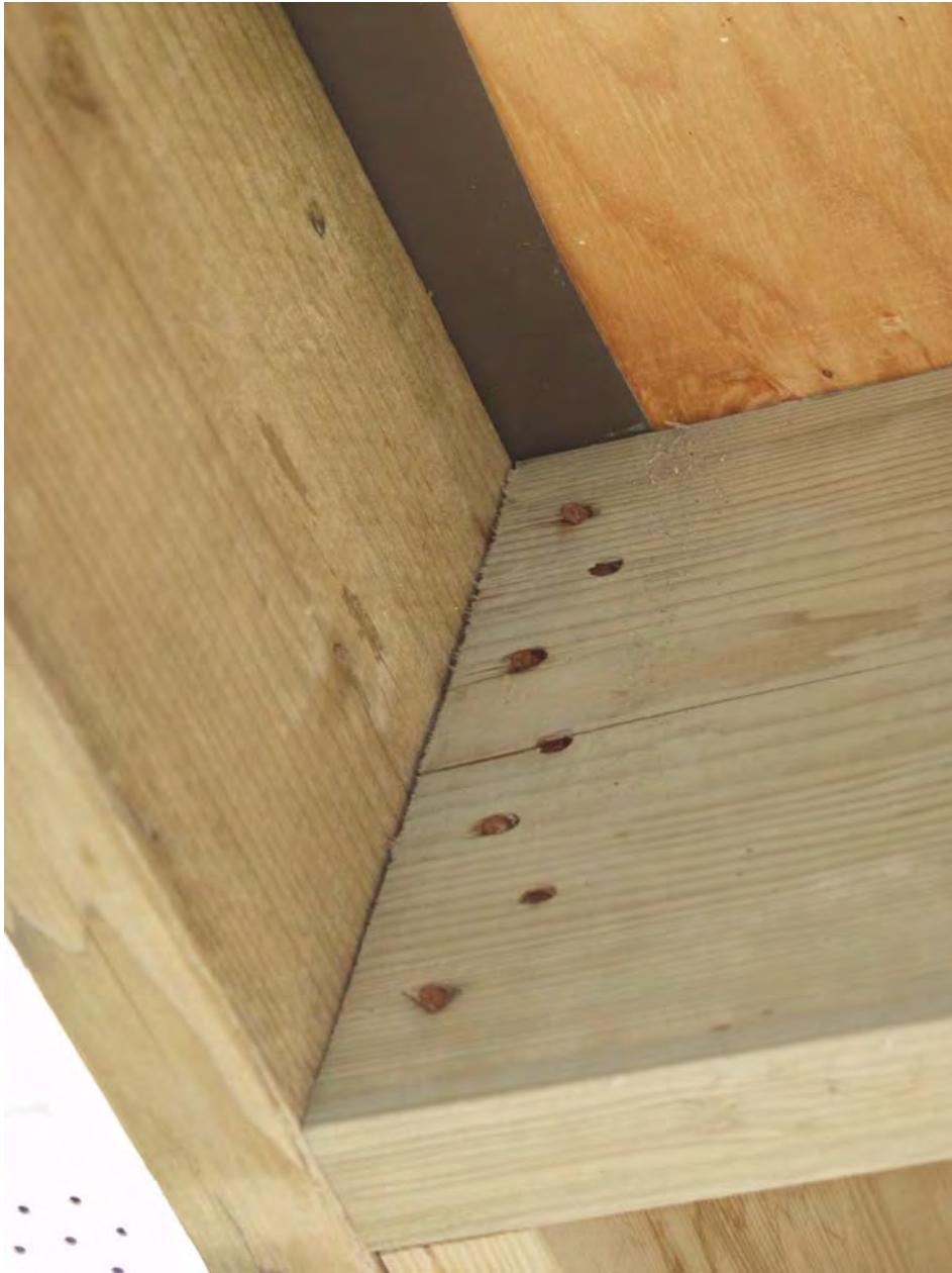
Figure 21. Red rust on common mild steel nails fastening deck joist to rim joist.
