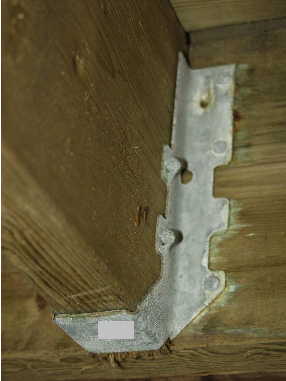
Figure 17 Small amount of red rust on the edge of proprietary hanger, (the specifications of which meets the G185 requirement)
