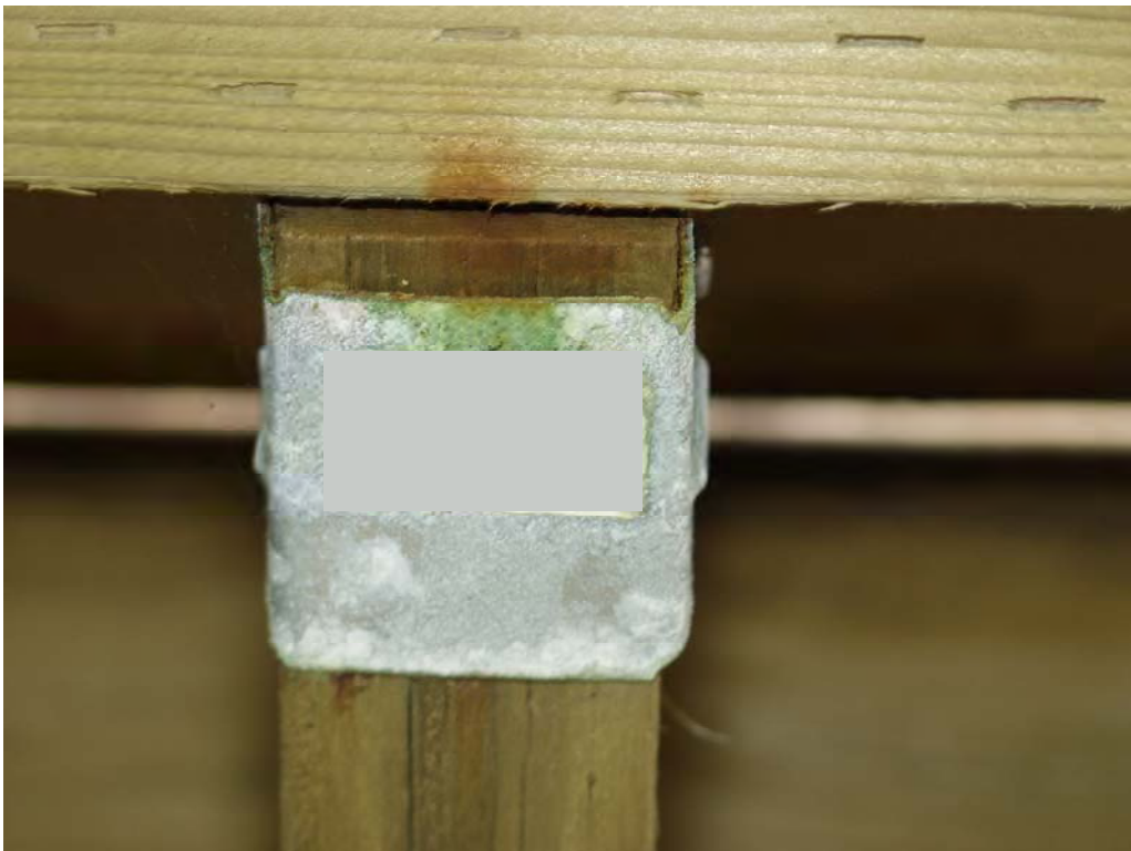
Figure 4 Hanger with red rust and copper deposits
