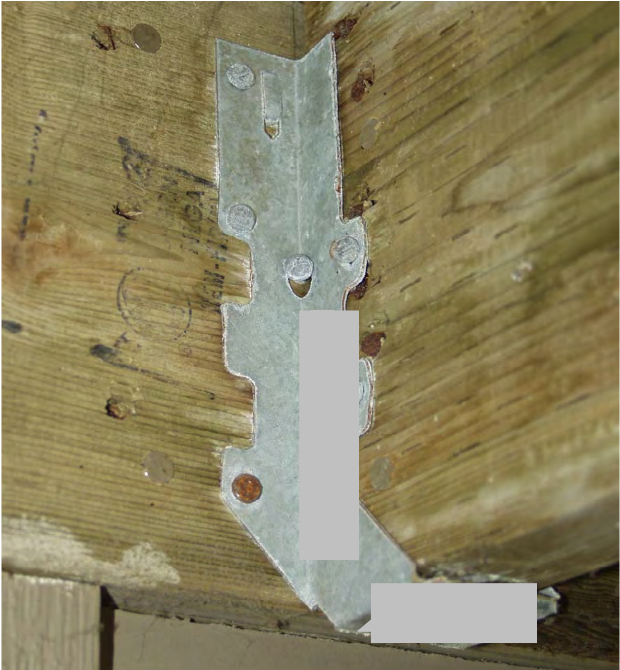
Figure 14 Small amount of red rust on edge of proprietary hanger, (the specifications of which meets the G185 requirement) and lower galvanized nail head. Common nails on right have red rust.
