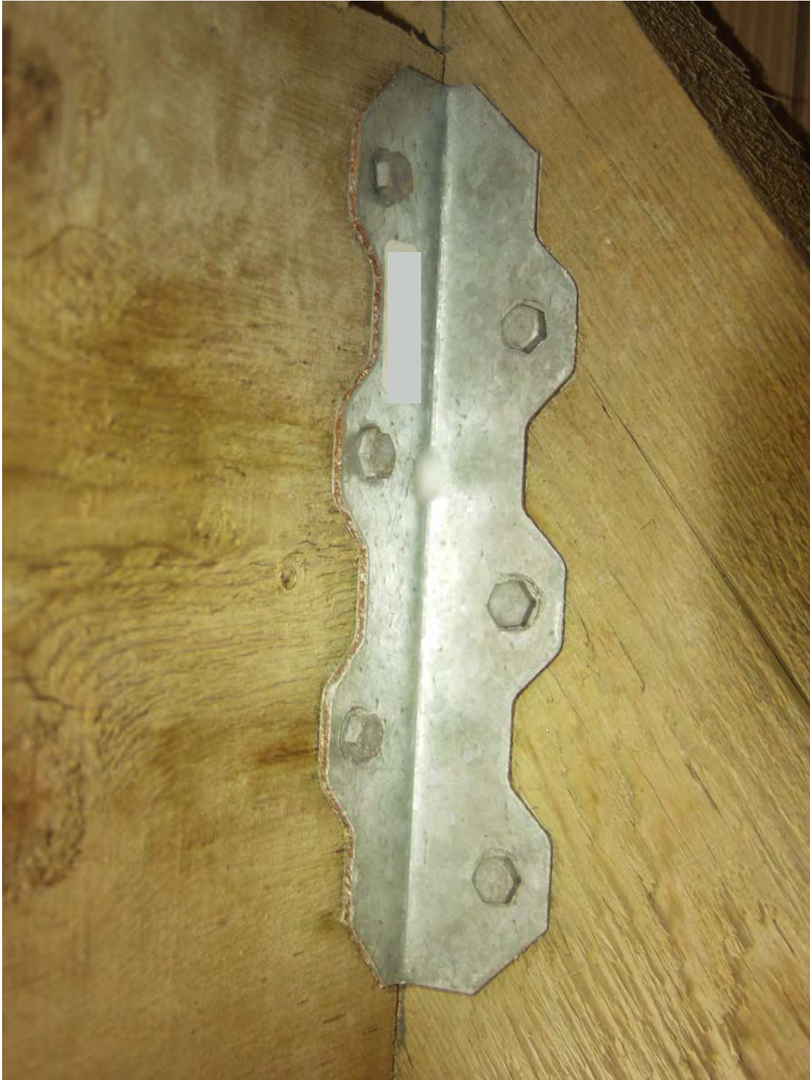
Figure 46. Galvanized connectors showing red rust on the edge. Note lack of copper deposits on wood and lack of corrosion on face.
