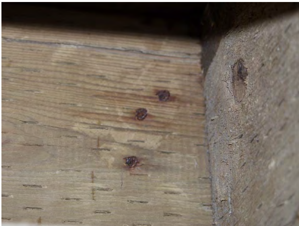
Figure 8 Corrosion of mild steel un-galvanized nails
