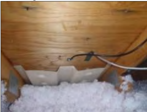
Figure B.11: Unit 2 west baffle
