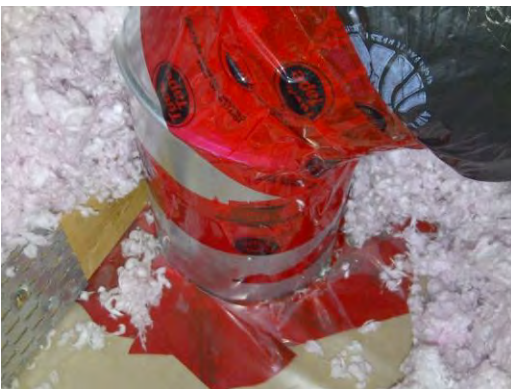
Photo 6: Air Barrier Sealing of Dryer Duct Penetration at Ceiling
