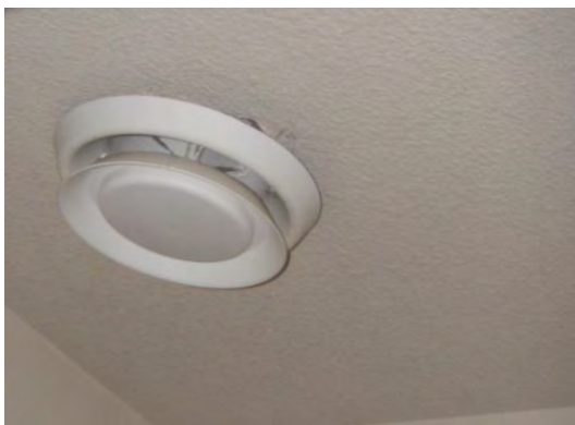
Photo 10: Fresh Air Grill with Air Leakage Path
