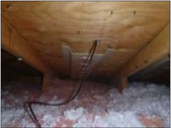
Figure B.27: Unit 4 south baffle
