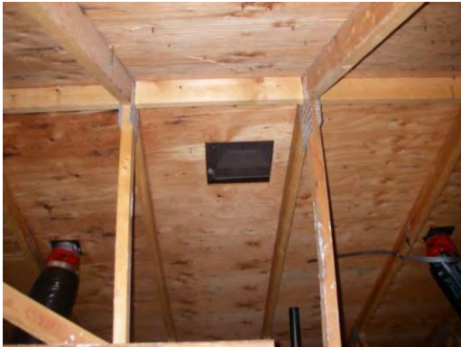
Photo 4: Roof Penetrations and Vent at Ridge
