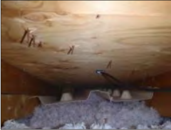
Figure B.17: Unit 3 east baffle
