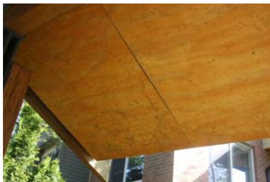
Photo 1: mold growth on the plywood cover below the sensor locations for the control roof assembly. This mold growth is after two winters exposed to ambient conditions at the study location.
