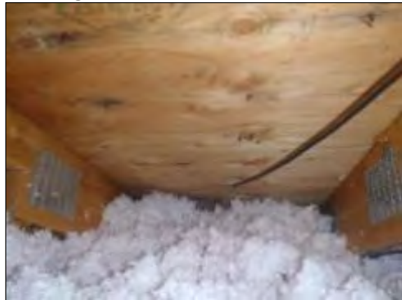
Figure B.4: Unit 1 west non-baffle
