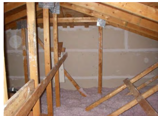
Photo 9: Drywall Fire Separation
