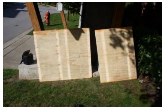
Photo 2: staining of the backside of the plywood cover. Notice at the location where the plywood was in contact with the rafters is clean.
