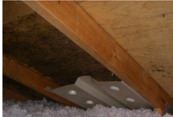
Photo 5: Baffle Vent at Soffit
