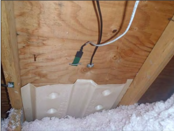
Figure B.25: Unit 4 north baffle
