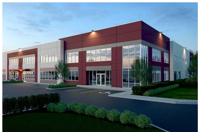
Figure 5: Example of a Retail Building (Source: REA)
