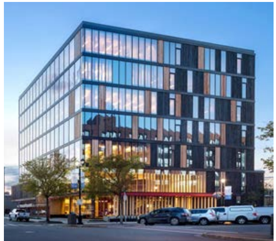
Figure 4: Example of a Commercial Office Building (Source: MGA)
