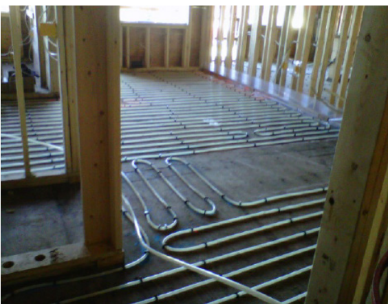
Rose Harbour. In-floor radiant heating
