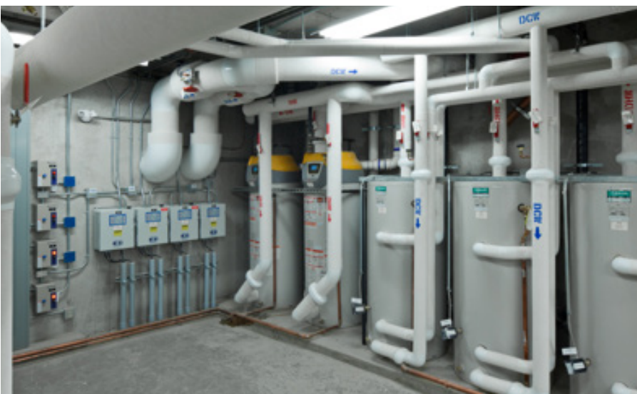
1005 Station Street, Vancouver. 80 units - 6-storey building. Mechanical room
