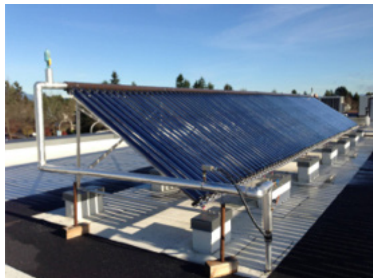
Alexander Street. 139 units - 7 storeys. Solar system re-commissioning
