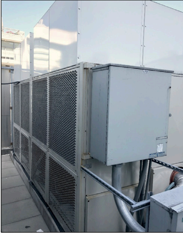
1249 Howe St. Air-to-water heat pump chiller. ATHP-1 - Airstack ASP 060X-H (2 modules)
