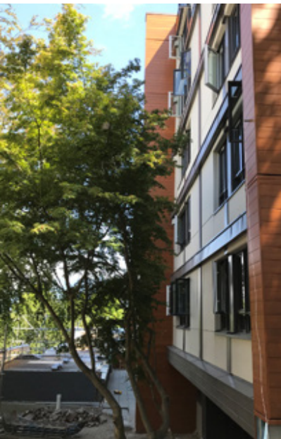
Grandview Terrace. Building envelope upgrade
