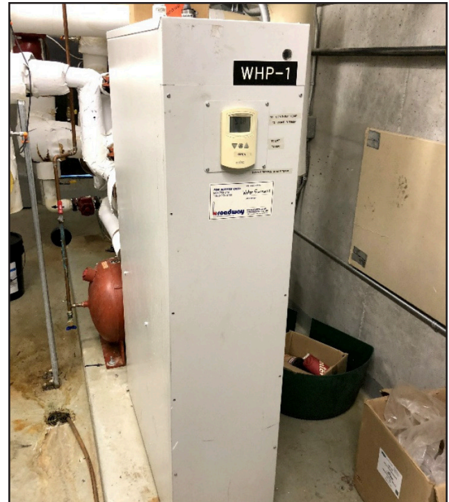
1249 Howe St. Water-to-water heat pump WHP-1
