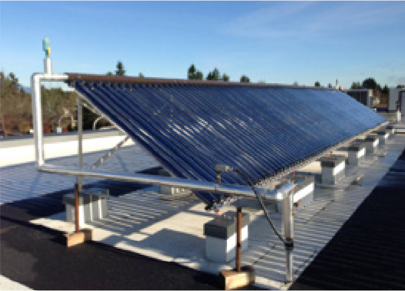
Alder Gardens. 36 units - 4-storey wood frame apartment with 1-level underground parking. Solar domestic hot water heating
