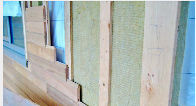
Vertical wood strapping mounted outboard of exterior insulation, attached to wall with long screws.
