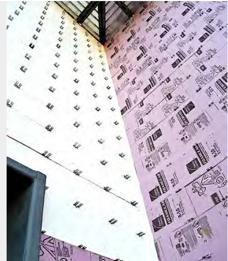
Galvanized steel clips support exterior insulation and cladding.
