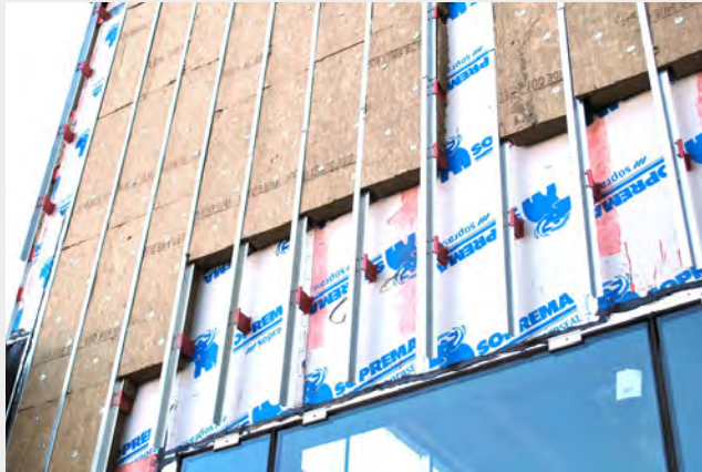
Z-girts flush with face of exterior insulation, mounted to wall with low conductivity stand-off clips.
