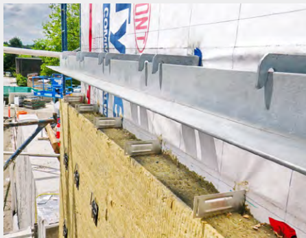
Stainless steel masonry ties and stand-off ledger angle support for brick.
