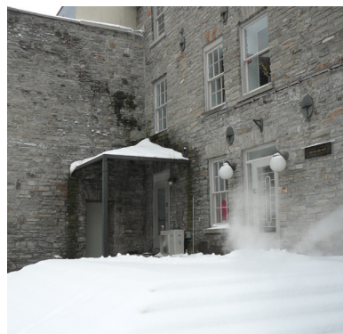
Moisture from flue gases accumulating on the wall of a heritage building will affect the durability of that building.
