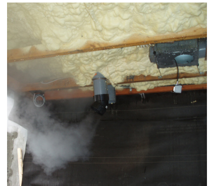
Venting should never be placed underneath the building or cold floor areas.
