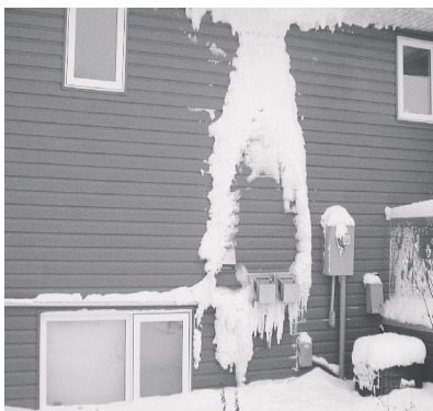
In cold climate conditions, vent gas condensation is visible as frost buildup against wall and roof overhang.
