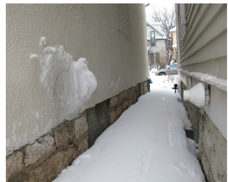
Sidewall vented appliance retrofitted into an older home blows flue gases against the neighbouring house where it has led to ice buildup.
