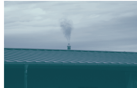
Furnace flue gases from a high efficiency furnace vented through the roof – mostly moisture.
