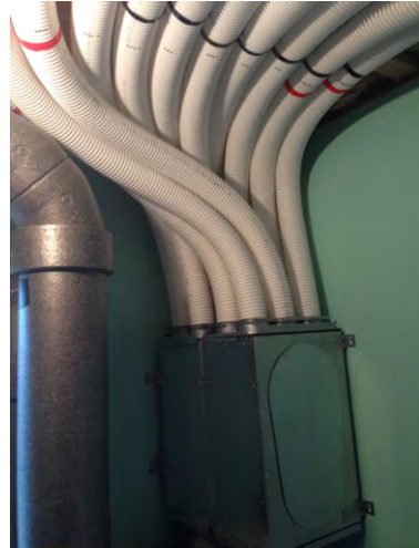
Figure 5: Mixing box (HRV not shown), with home-run ducting (HDPE with smooth interior surface). Image courtesy of NZ Builders.
