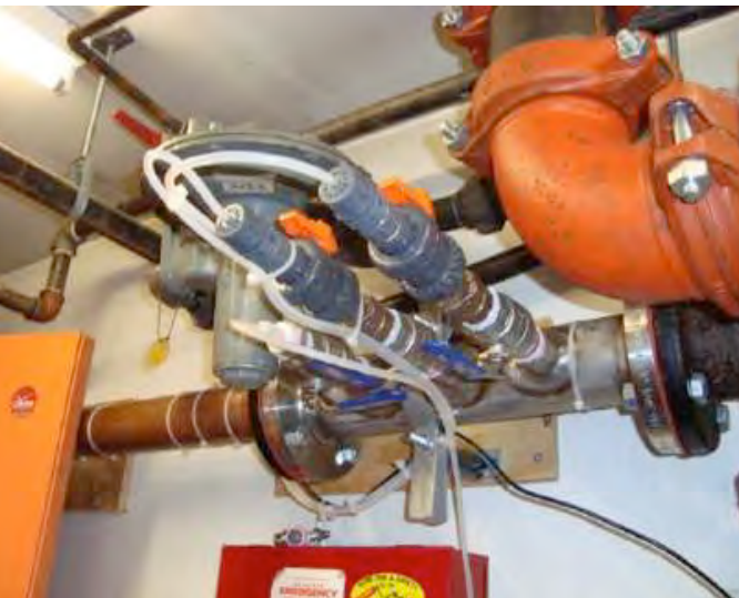
Image of the injection point of minerals into the domestic cold water supply.
