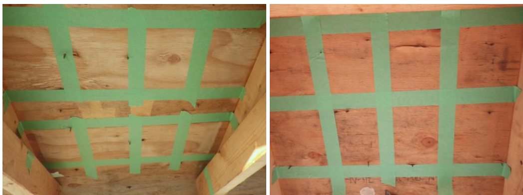
Figure 2.2 The sanded surface (left) and the existing unsanded surface (right) on the underside of the 3:12 North roof sheathing prior to treatment
