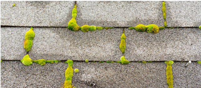
An accumulation of moss will tend to hold moisture on the roof, preventing proper drainage and accelerating the deterioration of roofing components.
