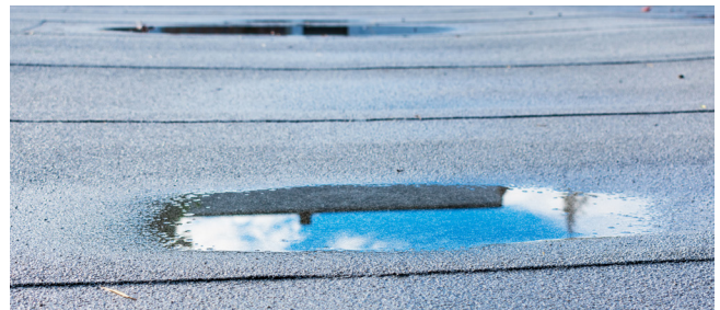
A large blister on this two-ply, low-slope roof has caused the membrane to move at the seam. The membrane has split under this stress and the blister is now full of water.
