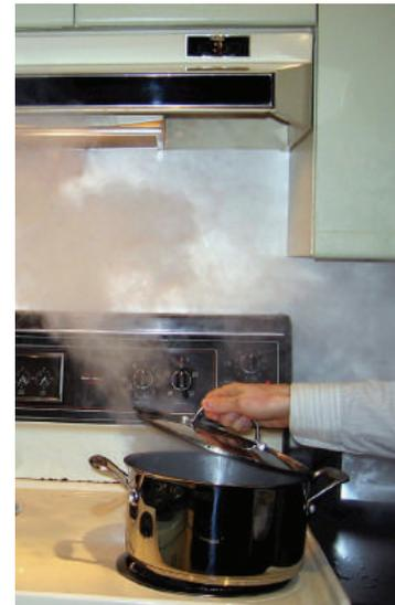
Use your kitchen exhaust fan or range hood to remove humidity generated by cooking. The exhaust fan should be vented to the outside.
