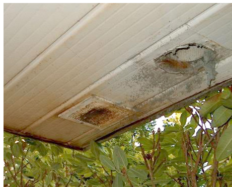
The build-up of debris or dirt on the underside of the balcony limited the air flow through the vent, resulting in damage.
