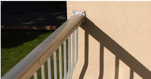
Guardrail connection to the wall can be a vulnerable point of water ingress.
