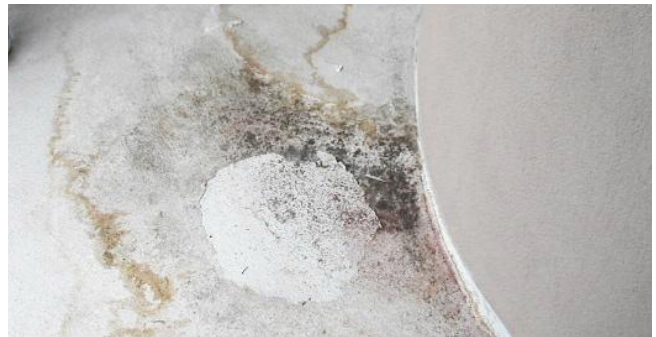
Staining on this deck membrane indicates ponding. Holes or punctures must be repaired as soon as possible to avoid water entering the structure when it rains.
