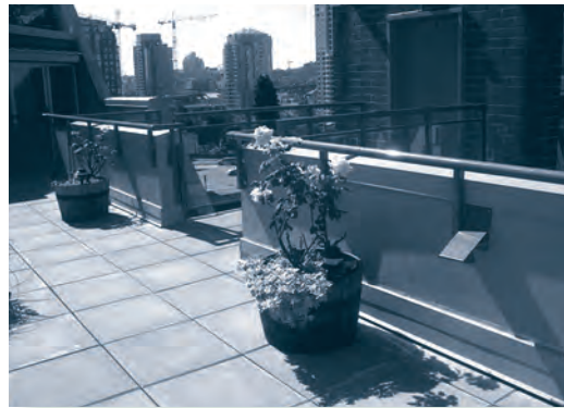
Deck with combination of guardwalls and guardrails.
