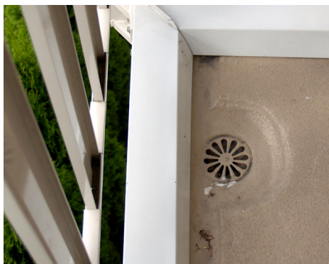
Maintain drains free of obstructions, dirt or debris to ensure they are free flowing and to prevent water ponding.
