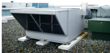
Typical rooftop make-up air unit
