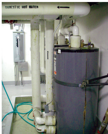
Central domestic hot water system
