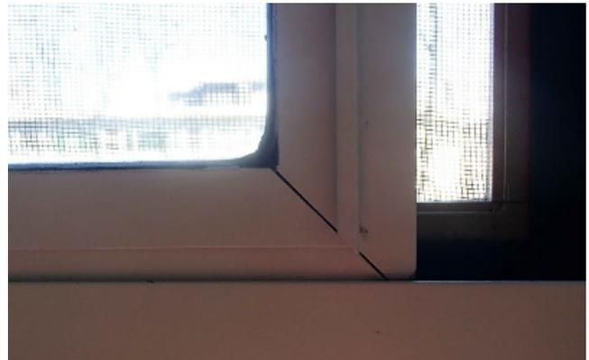
*Misaligned miter at the corner of aluminum window frame*
