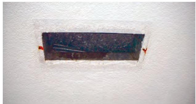
Indications of condensation build up.
