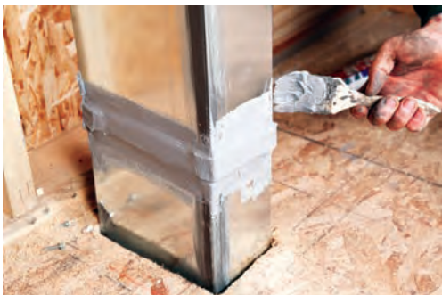
Duct sealing from the outside.
