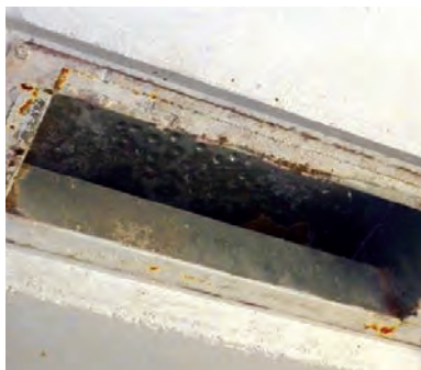
Indications of condensation build up.
