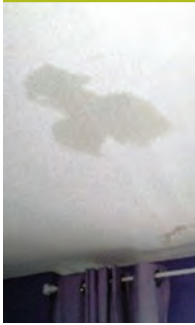
Poorly designed or unmaintained ducts can lead to damaged finishes from condensation build up.
