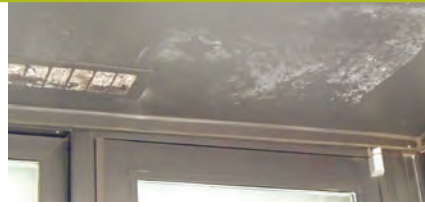
Poorly designed or unmaintained ducts can lead to damaged finishes from condensation build up.
