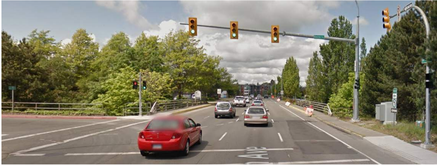
Vernon Avenue Existing Conditions
