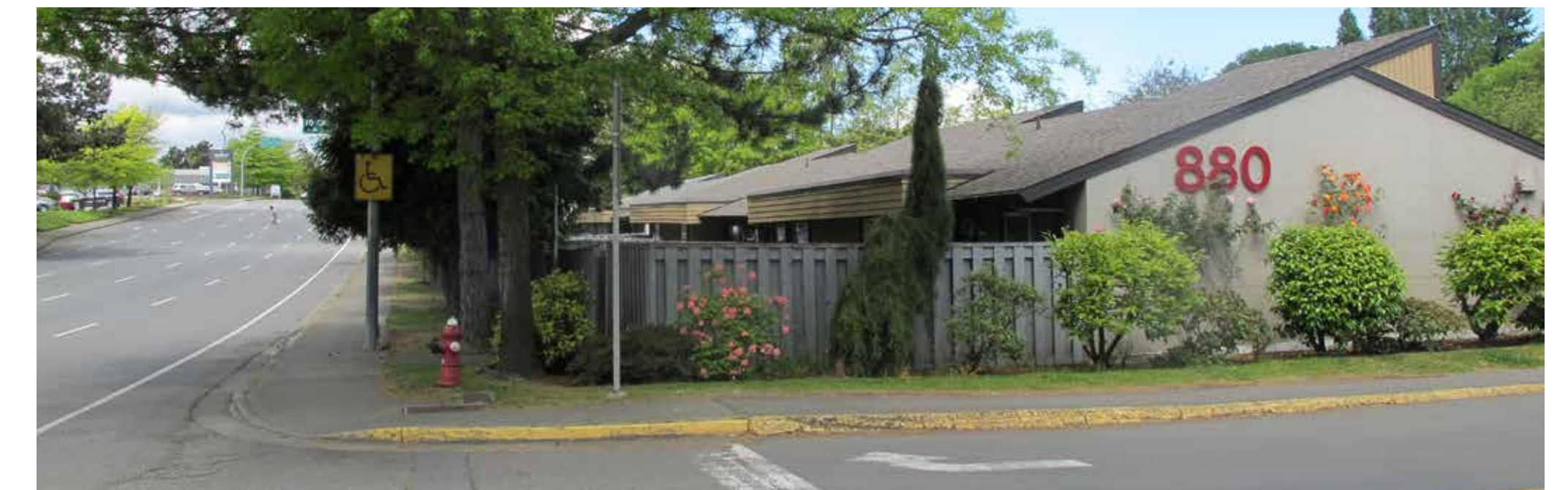
Access from Vernon Avenue
