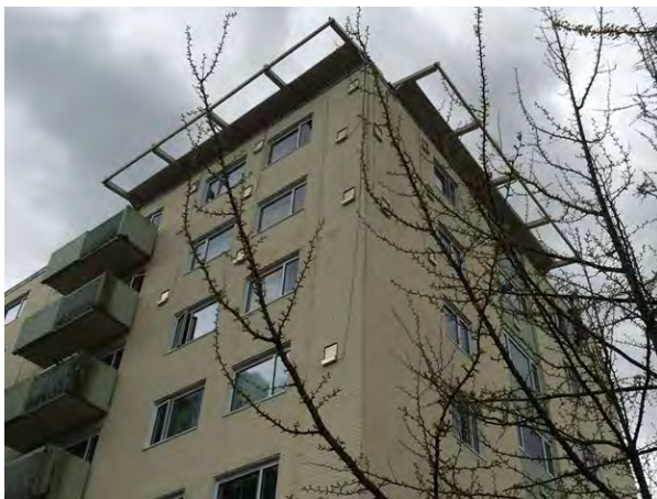
Figure 2: A 0.6-metre overhang.
