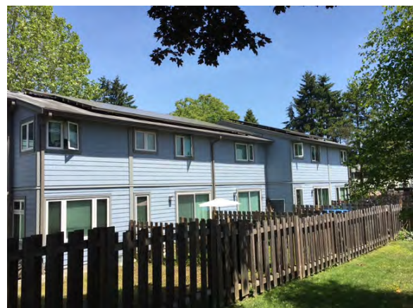
Figure 1: PV system installed at Greenbrook.
