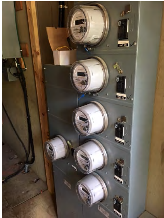
Figure 2: Electrical meters at Greenbrook.
