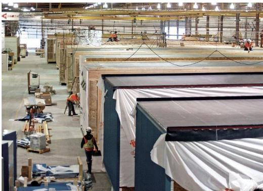
Figure 46 - When they are craned into place, the modules for TWU were about 95% complete. (© Metric Modular)
