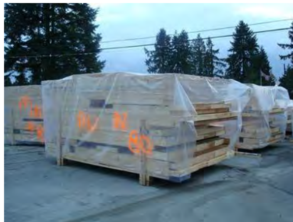
Figure 9 Covered prefabricated framing at a construction site
