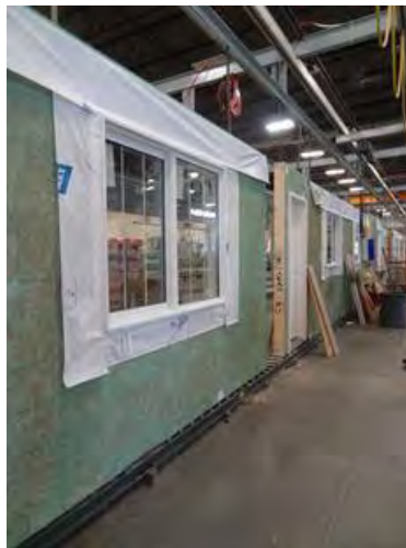
Figure 2 Prefabrication of building assemblies in a factory
