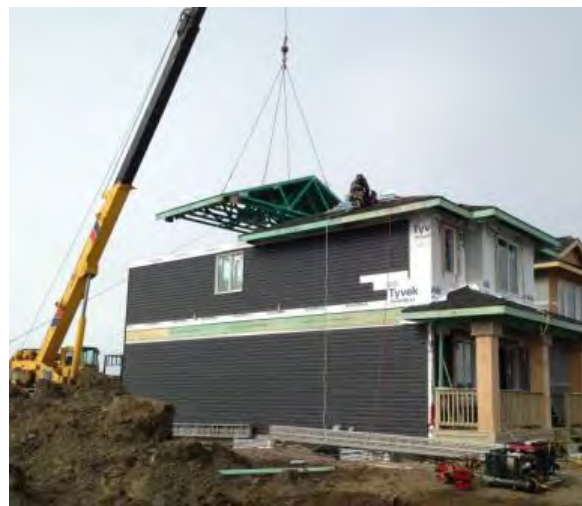
Figure 8 Installing a modular roof on a house
