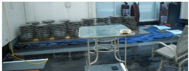
Stacked concrete pavers during membrane repair work
