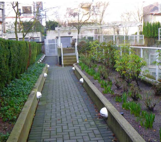
A typical courtyard at-grade assembly. This courtyard features many different types of overburden, making access to the underlying membrane difficult.
