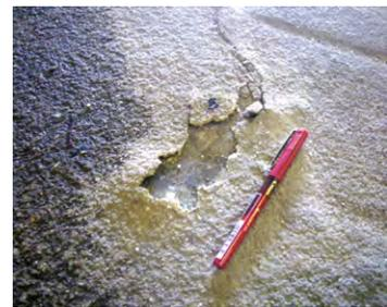
Delamination of suspended concrete slab membrane.
