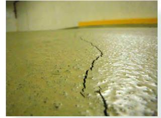
Cracks in a suspended concrete slab membrane.
