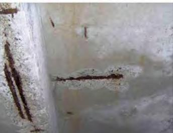
Corroding reinforcing steel and delaminated concrete.
