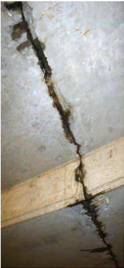
Water ingress through a crack in the concrete slab.
