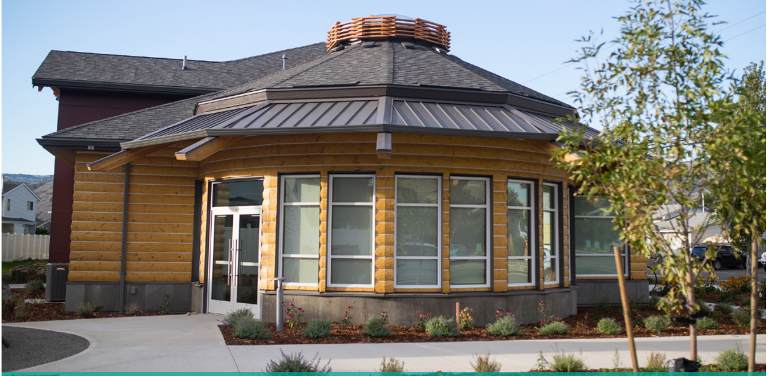
Kee-Kek-Yel-c in Kamloops, built to BC Energy Step Code Level 3 and opened in September 2020.
