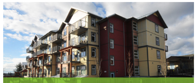
Photo: Rosalie's Village, Vancouver Island, a LEED certified building opened in March 2017
