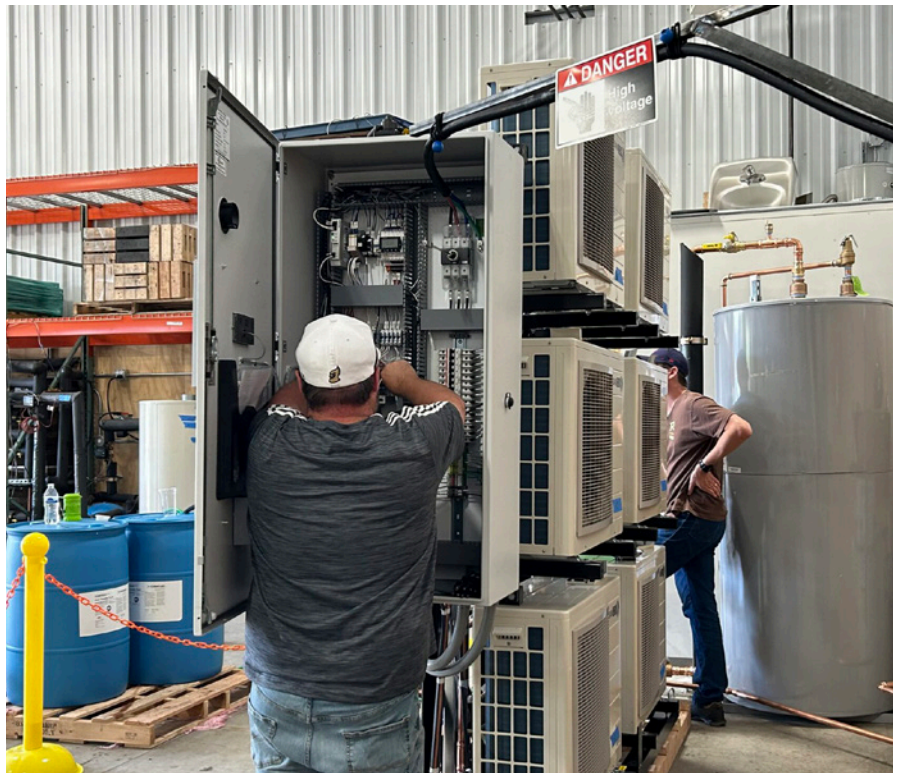
An engineer works on the electrical and control panel for one of three Vienna House Droplet hot water plants. (Source: Viennahouse.ca)
