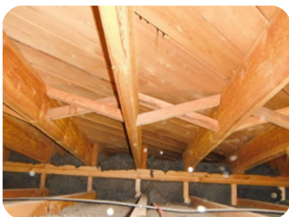
Figure 5: Range of observed low-slope vented wood-framed roof sheathing conditions in the Lower Mainland of BC at time of roof membrane renewal
