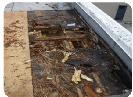
Figure 5: Range of observed low-slope vented wood-framed roof sheathing conditions in the Lower Mainland of BC at time of roof membrane renewal
