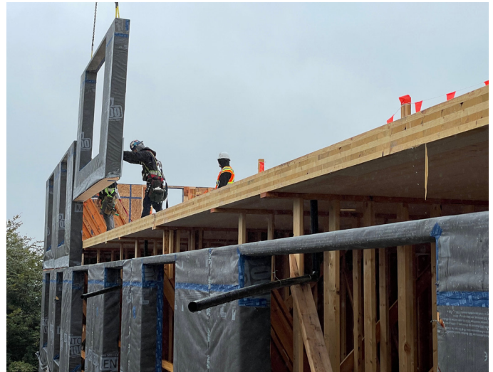
Figure 4. Installation of exterior wall panels (source: Scius)
