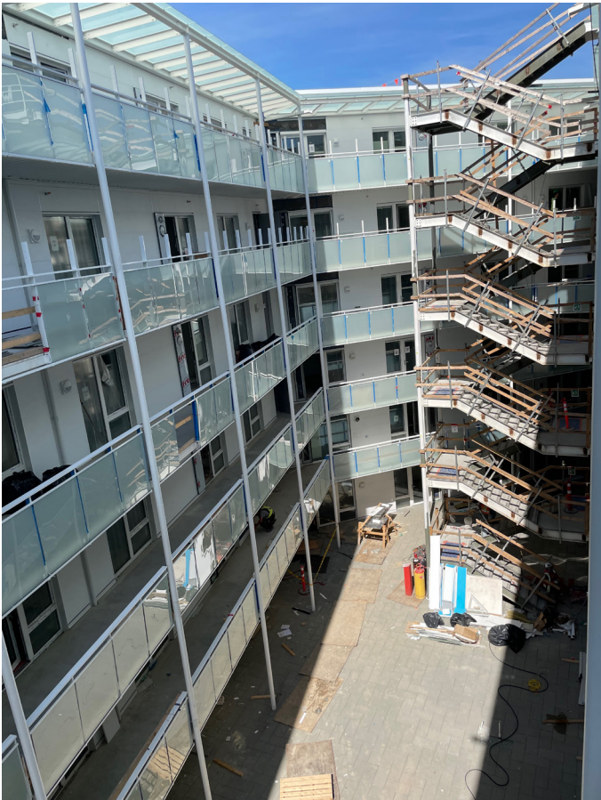
Figure 3. The courtyard at Vienna House, under construction May 2026 (source: Scius)
