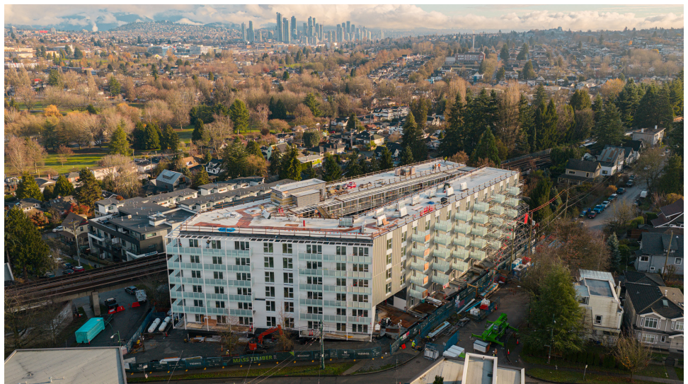
Figure 1. Vienna House during construction, December 2025 (source: Kindred Construction)
