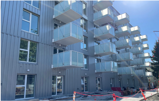
Figure 12. Balconies along the south side of Vienna House (source: Scius)
