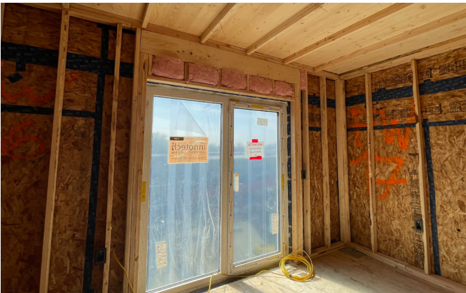
Figure 7. Another suite with interior of double-stud framing completed and second layer of insulation partially installed. (source: Scius)
