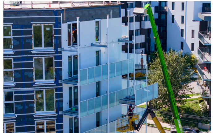
Figure 15. Installation of large balconies (source: Kindred Construction)
