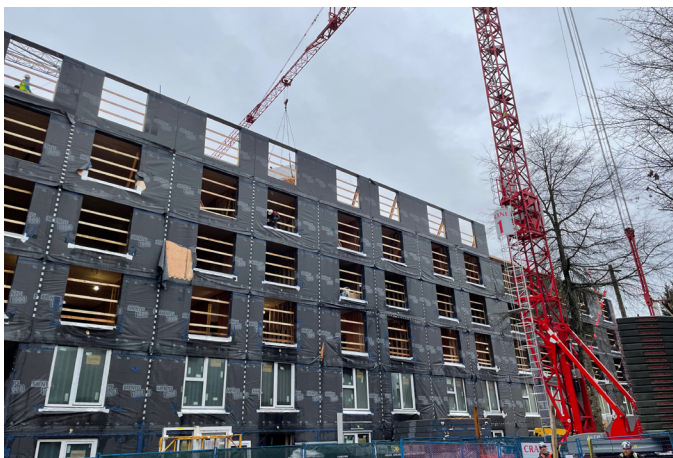
Figure 10. Crane 1 lifting a palette of panels onto Level 7. (source: Scius)
