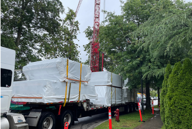
Figure 9. Panels arriving at Vienna House after transportation from Squamish (source: Scius)
