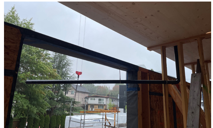
Figure 12. Water being routed to the exterior of the building with a temporary drain (source: Scius)
