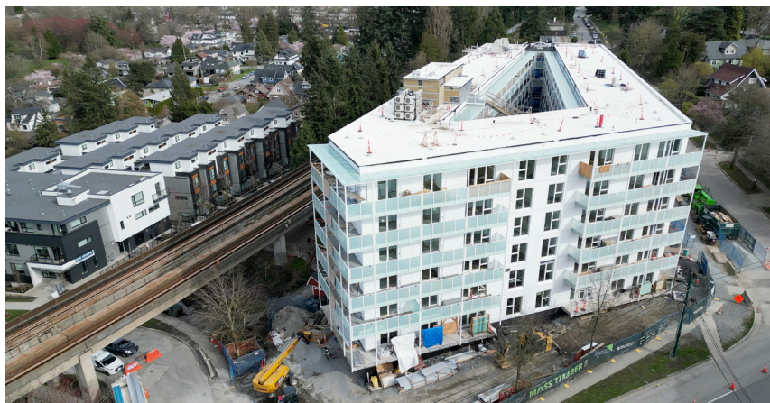
Figure 1. Vienna House during construction, April 2026 (source: Bright Future Studio)
