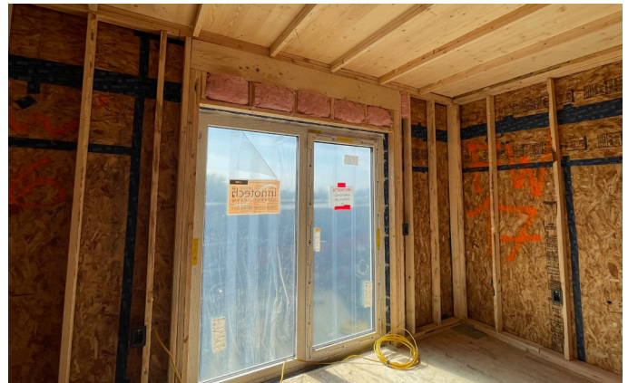
Figure 5. Another suite with interior of double-stud framing completed and second layer of insulation partially installed. (source: Scius)
