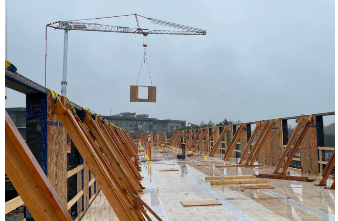
Figure 11. Exterior wall panels being installed (source: Scius)
