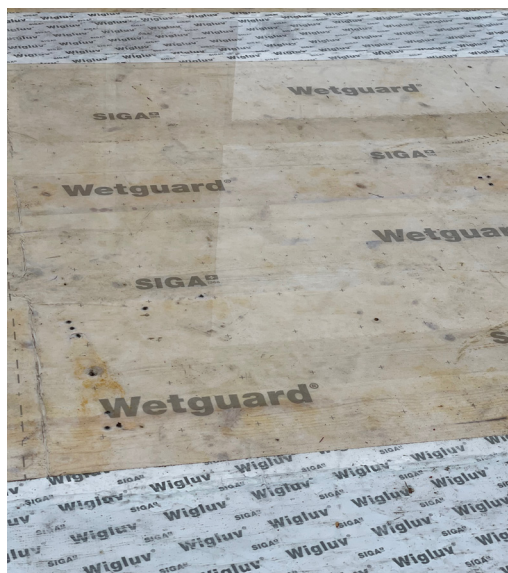
Figure 10. A weather protection membrane and taping on the top of installed CLT panels (source: Scius)
