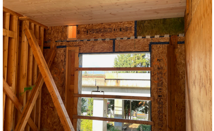
Figure 4. Interior of a suite with wall panel for above level attached. (source: Scius)
