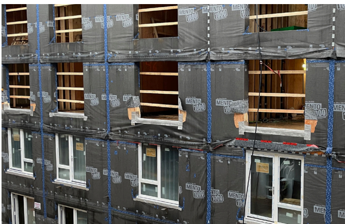
Figure 18. Preparations for window installation (source: Scius)
