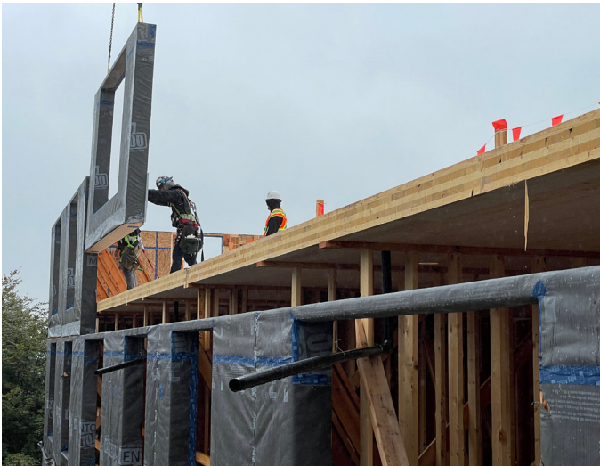
Figure 2. Installation of exterior wall panels (source: Scius)
