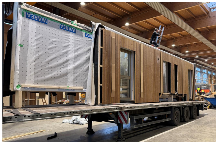
Figure 7. A wall panel at the factory loaded for delivery in Vienna, Austria (source: Rüdiger Lainer + Partner)
