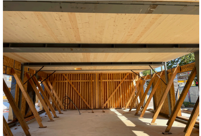
Figure 11. Steel, Prefab Walls and CLT were coordinated for construction of the amenity room (photo: Scius)
