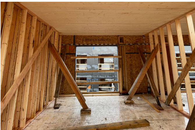
Figure 5. Prefabricated wall panels and CLT floor/ceiling. (photo: Scius)
