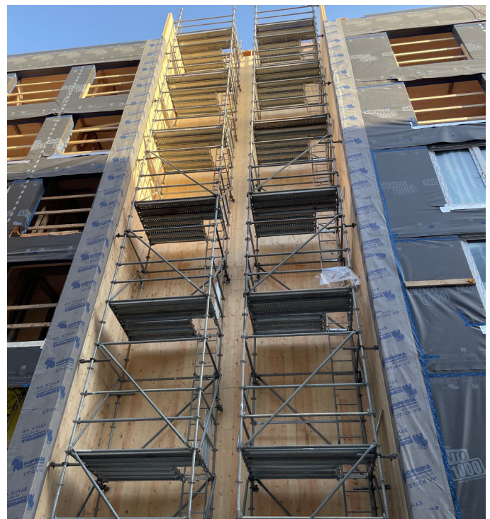
Figure 7. Details from the architectural and structural models were coordinated for the CLT elevator shaft. (photo: Scius)
