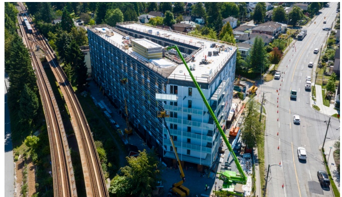
Figure 4. attaching balconies to Vienna House (photo: Kindred Construction)
