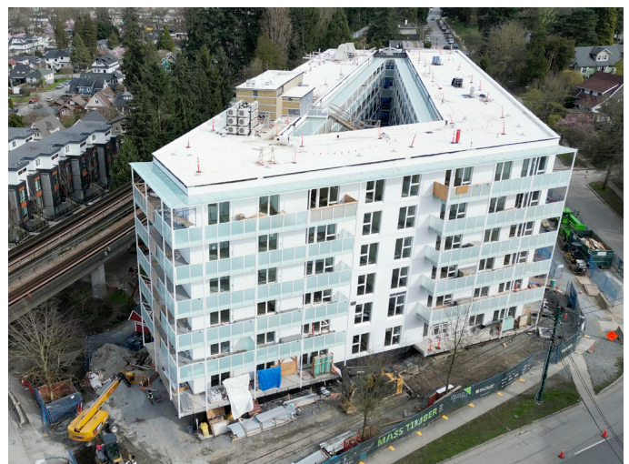
Figure 2. Vienna House under construction, April 2026 (photo: Bright Future Studios)
