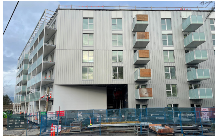
Figure 10. Vienna House under construction, January 2026 (photo: Scius)
