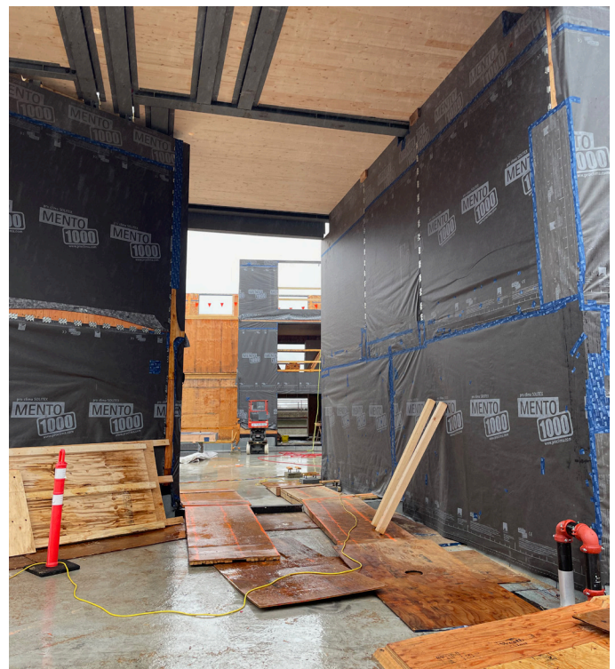
Figure 3. Vienna House under construction, September 2024 (photo: Scius)
