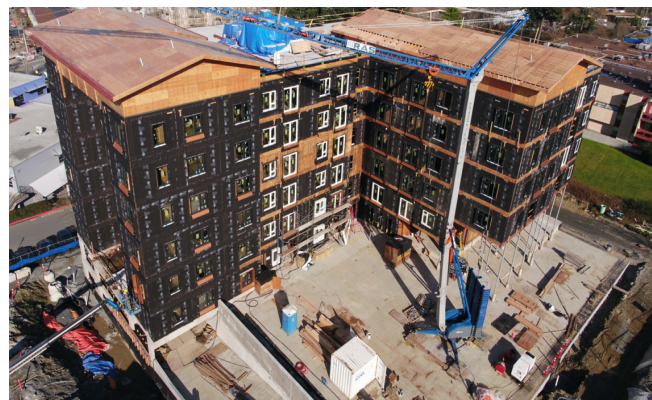
330 Goldstream utilized light-wood frame prefabrication.
