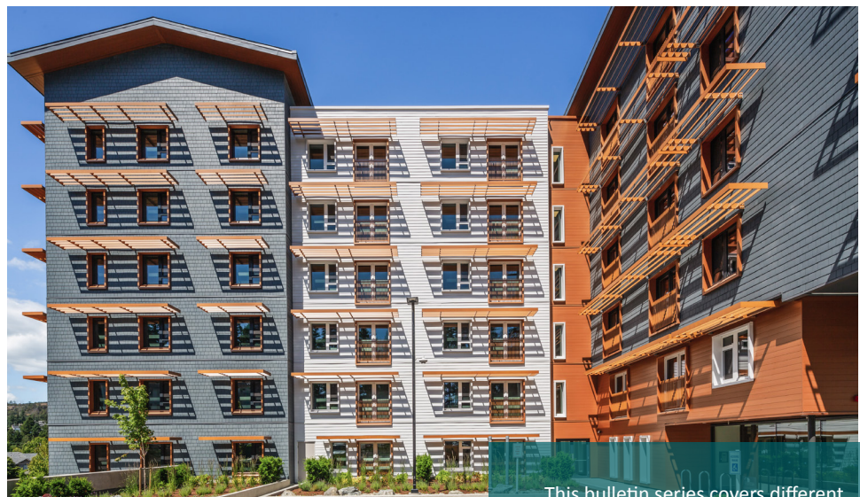
Completed 330 Goldstream Ave
