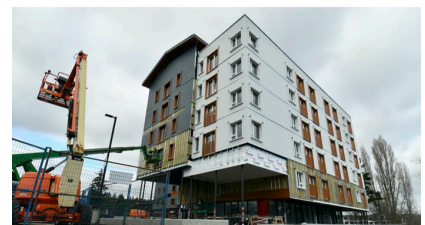
330 Goldstream under construction. Source: MultiVista
