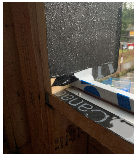
Tricky membrane flashing connections (Source: Scius)
