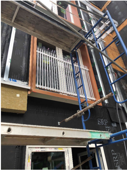
Image series: Complex flashing and cladding connections at building levels (Source: Scius)
