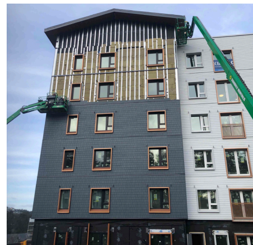
Brytar Contracting installing the cladding (Source: Multivista)
