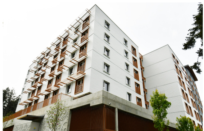
Parkade feature wall and large daylight portals. (Source: Multivista)
