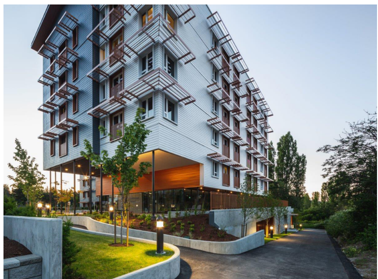
330 Goldstream provides direct access to the Galloping Goose Trail, which connects Colwood to neighboring municipalities, including Victoria. Photos courtesy James Jones in media publications & @jamesjonesphotos on Instagram
