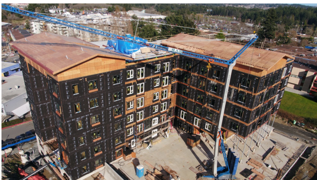
330 Goldstream utilized prefabricated light wood wall panels. (Source: Multivista)
