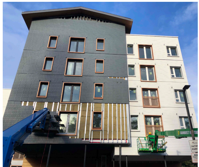
South Elevation, during construction.
