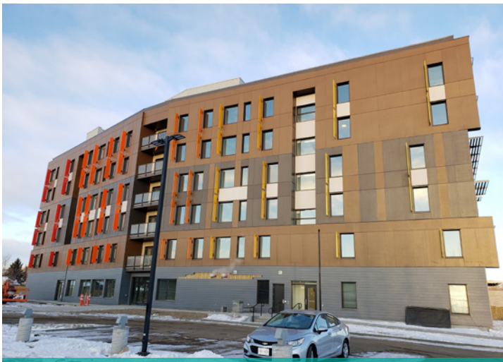
The Fort St John Multi-Family Passive House, certified to Passive House standards.
