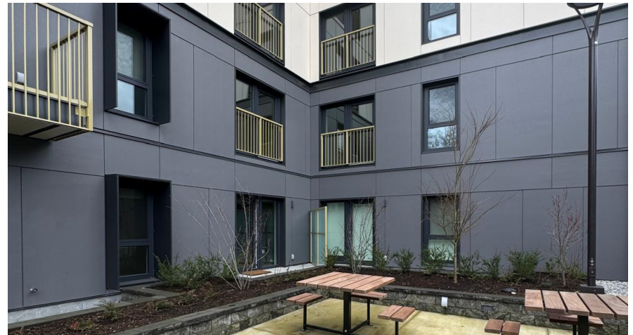
At Timbre & Harmony in Vancouver, there are both usable balconies and Juliette balconies. Image: Happy Cities
