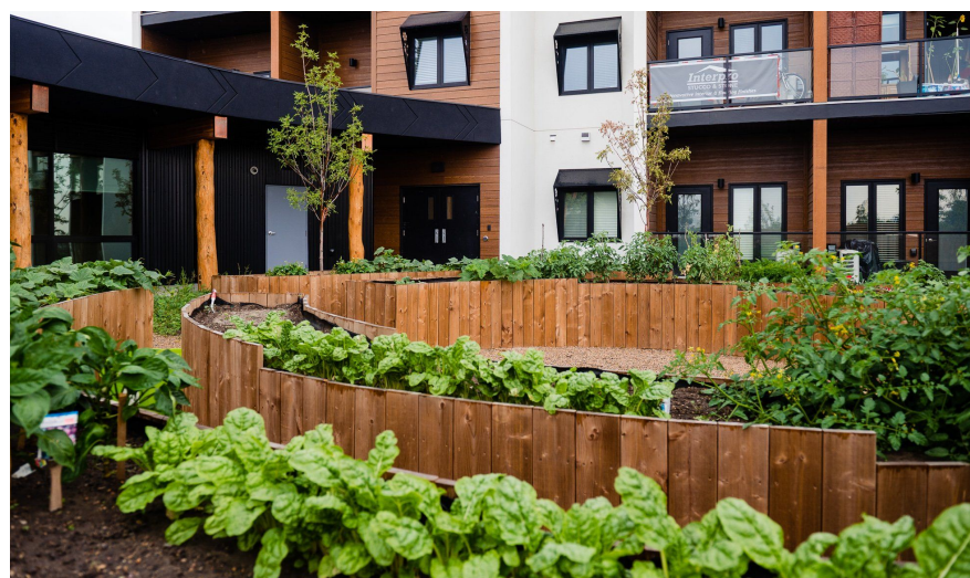
Round Prairie Elders' Lodge garden.. Image: David T. Fortin Architect / Big Block Construction
