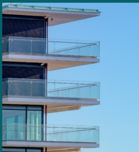
Figure 5. Cantilevered external balconies get a lot of attention as thermal bridges but less obvious thermal bridging at roof decks require equal consideration.
