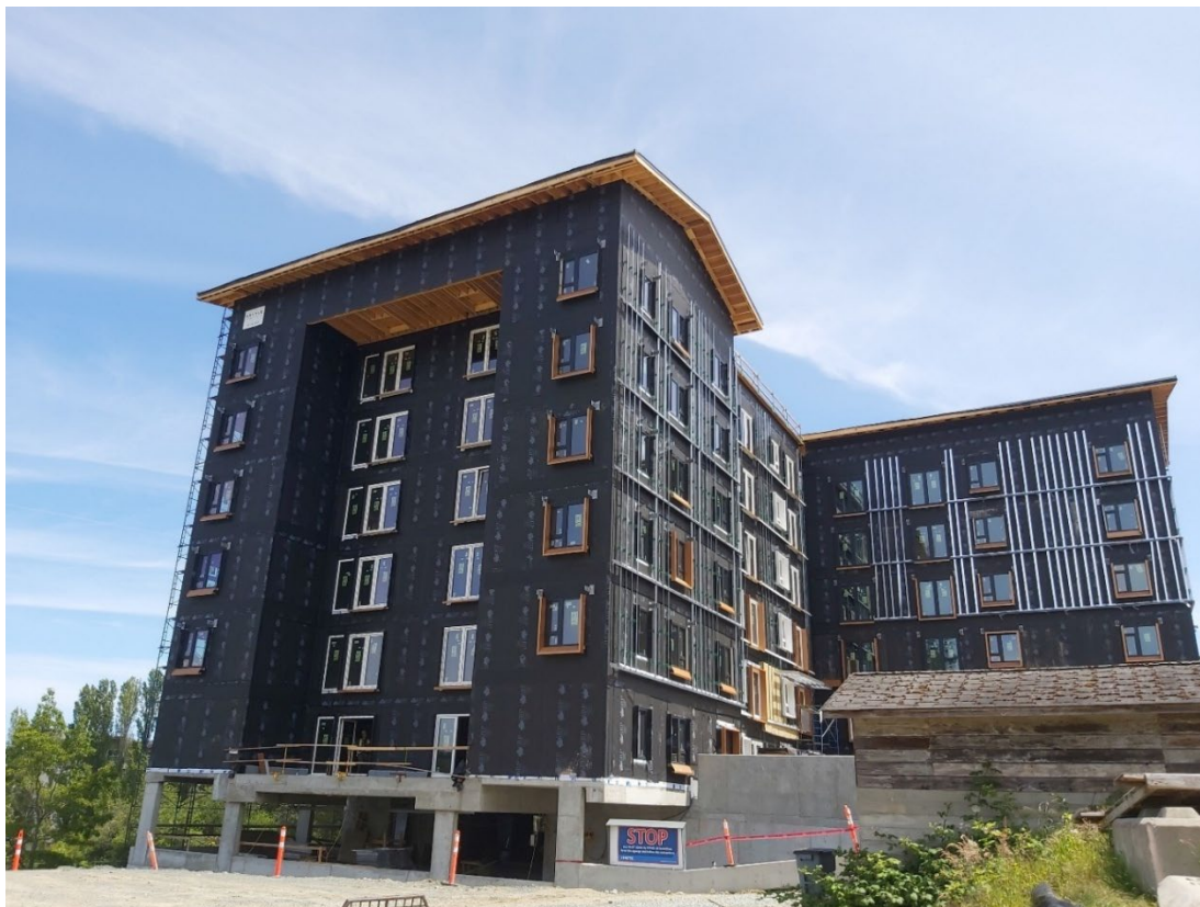
Figure 1. Building under construction.
