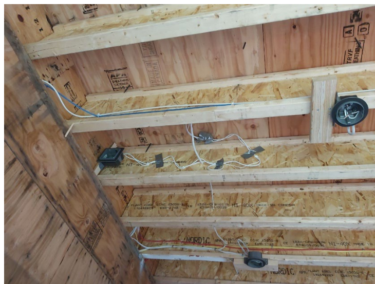
Figure 3. An RH/T/MC sensors with probes installed inside roof.
