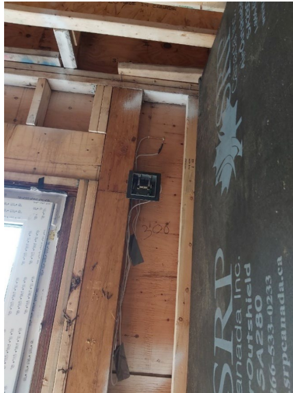
Figure 2. An RH/T/MC sensor with probes installed on interior surface of plywood wall sheathing.
