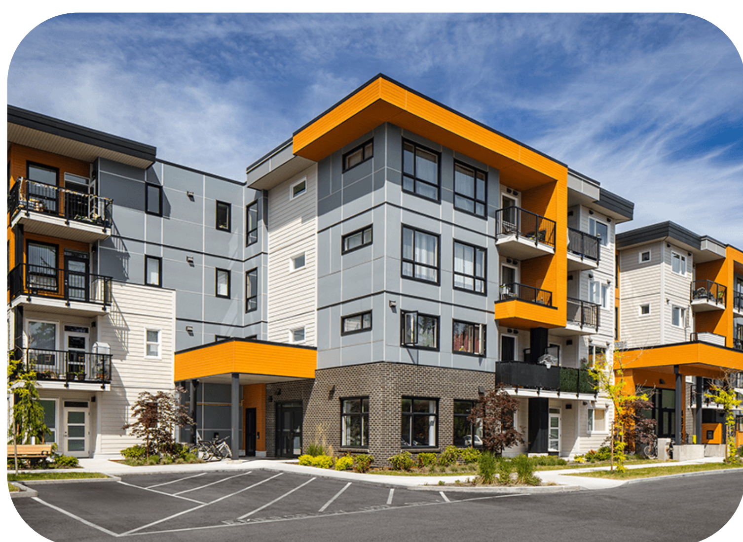
Tipton Place Affordable Rental Housing – 42 Units
