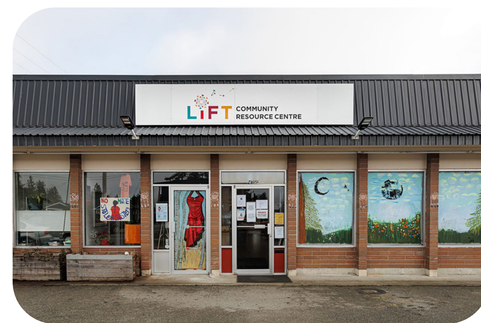
Lift Emergency Shelter Temporary Shelter – 20 spaces
