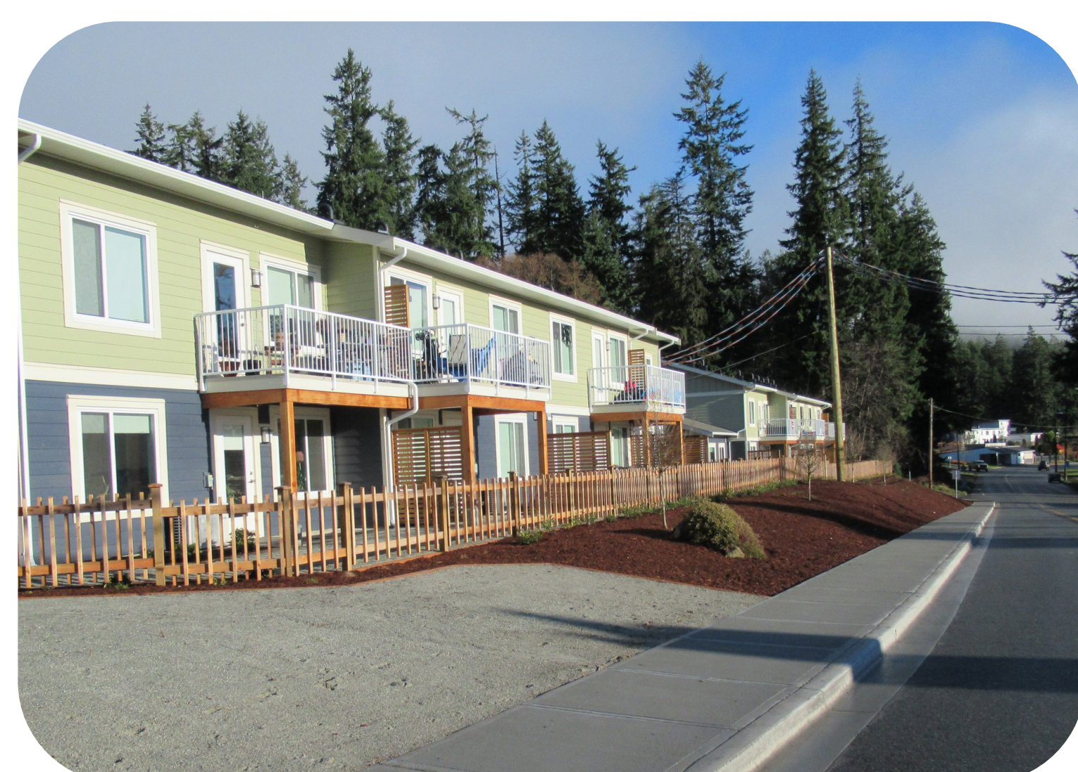
Cranberry Place Affordable Rental Housing – 24 Units
