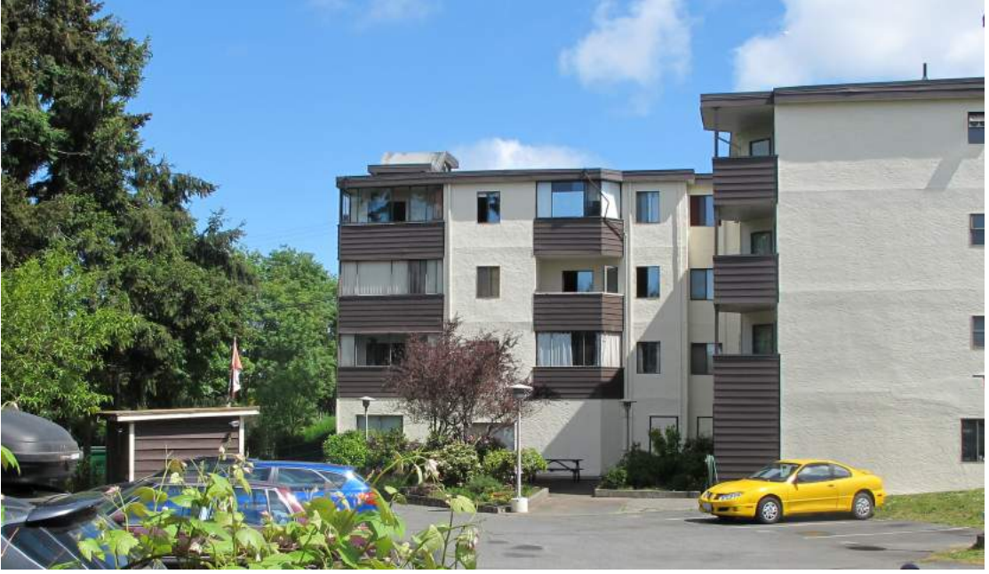
f. ICMH- Darwin Apartments
