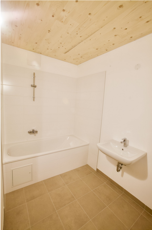
Figure 25. Washroom with CLT ceiling (source: Scius Advisory)
