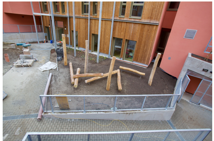
Figure 32. Play space under construction (source: Scius Advisory)
