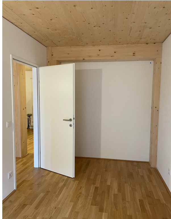
Figure 27. CLT ceiling and Glulam Beams in Bedroom (source: Scius Advisory)
