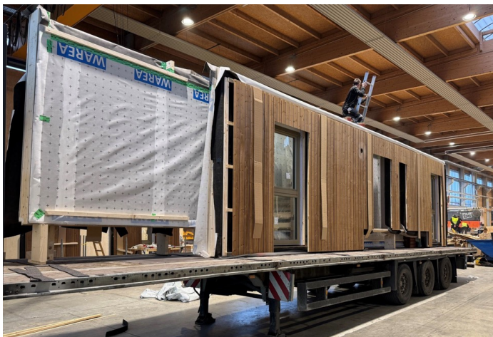
Figure 21. Exterior wall panels loaded onto a truck for delivery to Vancouver House. (source: Rüdiger Lainer + Partner)
