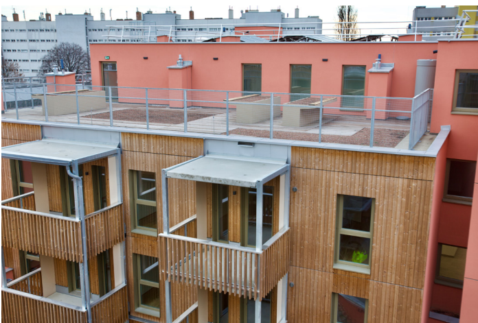
Figure 31. Planters on the rooftop of the assisted living building (source: Scius Advisory)
