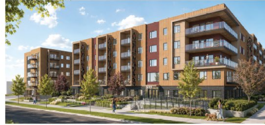
View of Building A from Georgia Avenue
