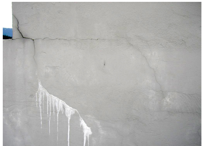
Water Penetration and Staining at Cracks
