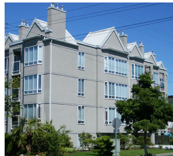
Typical four-storey, low-rise with rainscreen walls – Building 2 of the Monitoring Study. Flashing at each floor level directs water from the air cavity to the exterior and allows ventilation.
