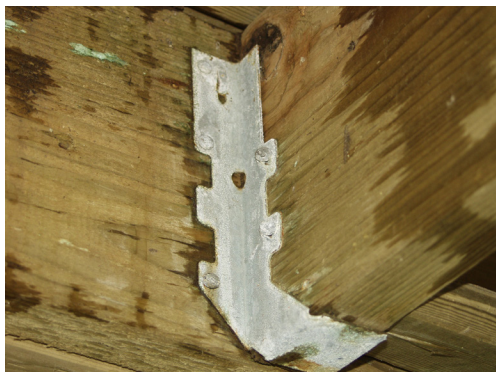
Only fasteners and connectors that are specifically recommended by manufacturers for use with alkaline copper treated wood should be used.
