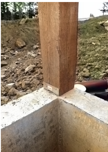
For structural components, stainless steel fasteners and connectors are recommended.
