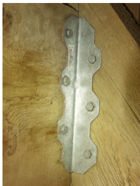
Only fasteners and connectors that are specifically recommended by manufacturers for use with alkaline copper treated wood should be used.
