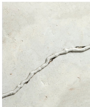
Crack filled with crack sealer
