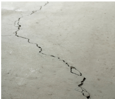
Typical concrete crack. Concrete driveway cracks may be covered under certain circumstances by home warranty coverage. It is advisable to consult the BC Housing Residential Construction Performance Guide for more details.
