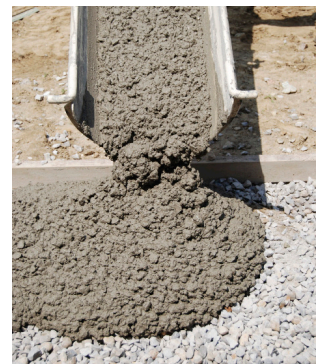
Concrete coming out of the chute onto graded gravel
