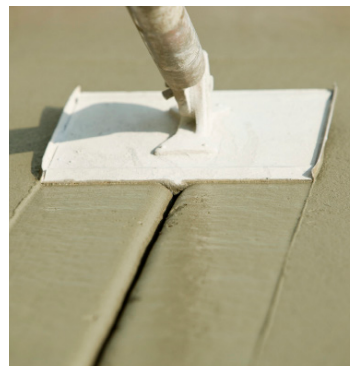
Adding a control joint to a freshly poured section of concrete.
