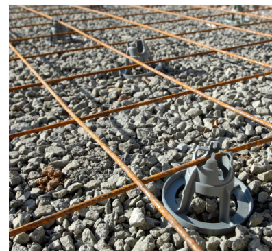
Foundation of a driveway before pouring the concrete.
